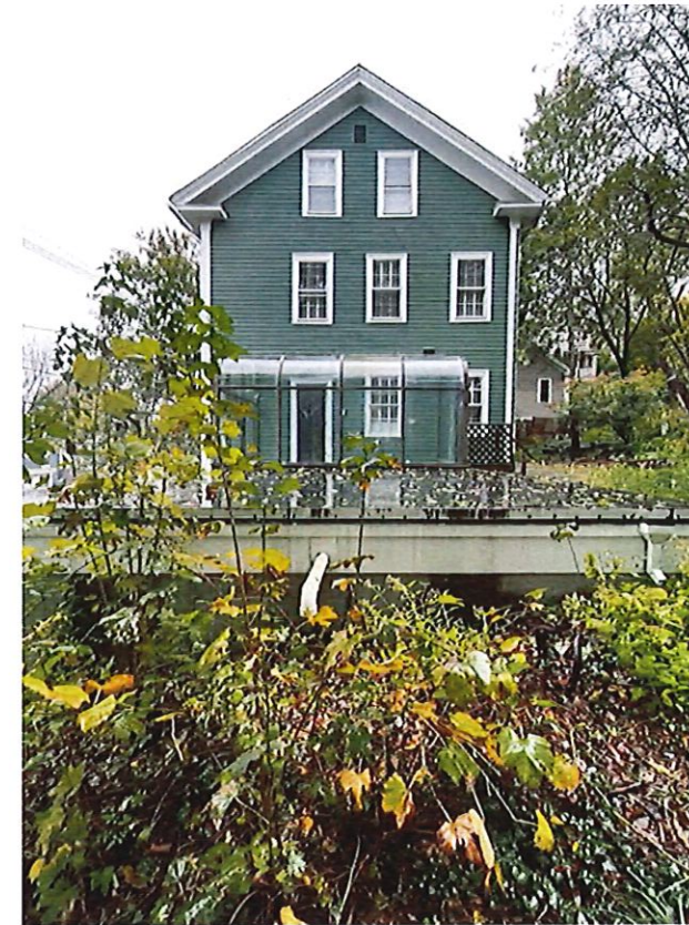
3 EXISTING CONDITIONS: SOUTH 56 PRATT ST.
