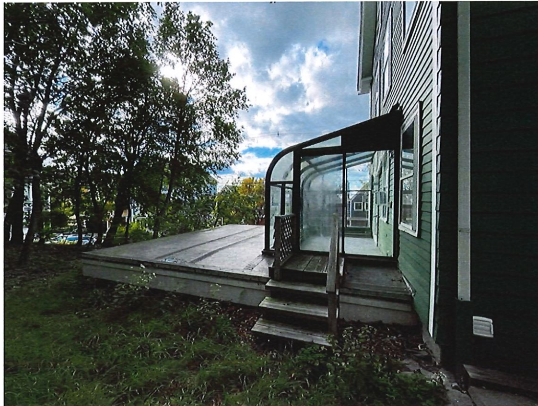
4 EXISTING CONDITIONS: EAST 56 PRATT ST.
