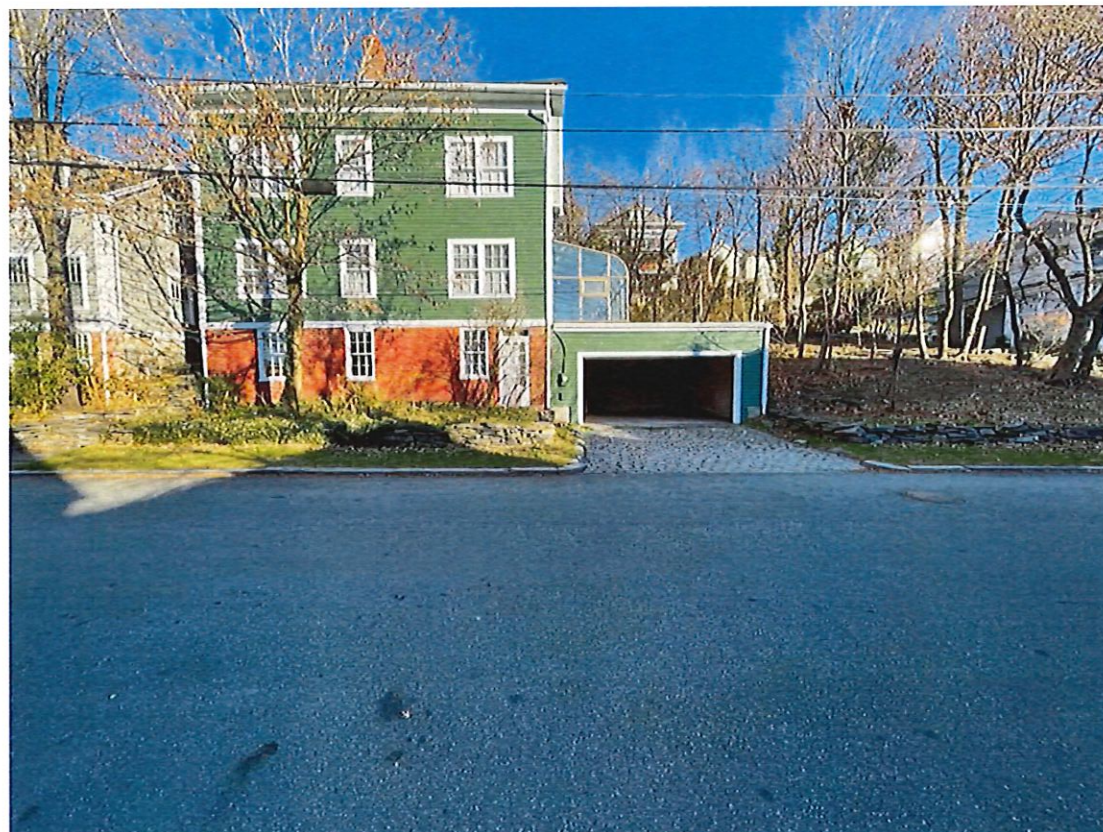
2 EXISTING CONDITIONS: WEST 56 PRATT ST.
