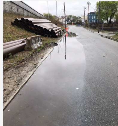
Broken Structures on Magnolia Street at Agnes Street
