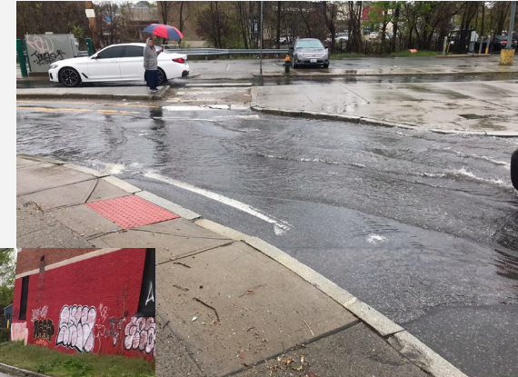
Clogged Structures at Hartford Avenue & Atwood Street
