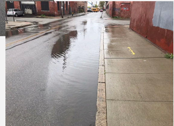
Clogged Structure on Troy Street at Oak Street
