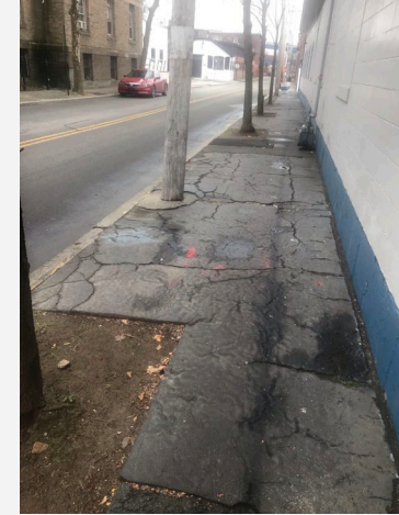
Non-compliant sidewalk along Troy St
