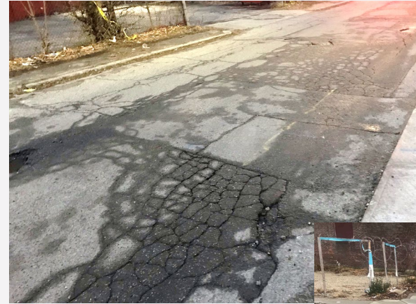
Alligator cracking along Atwood St next to Family Dollar
