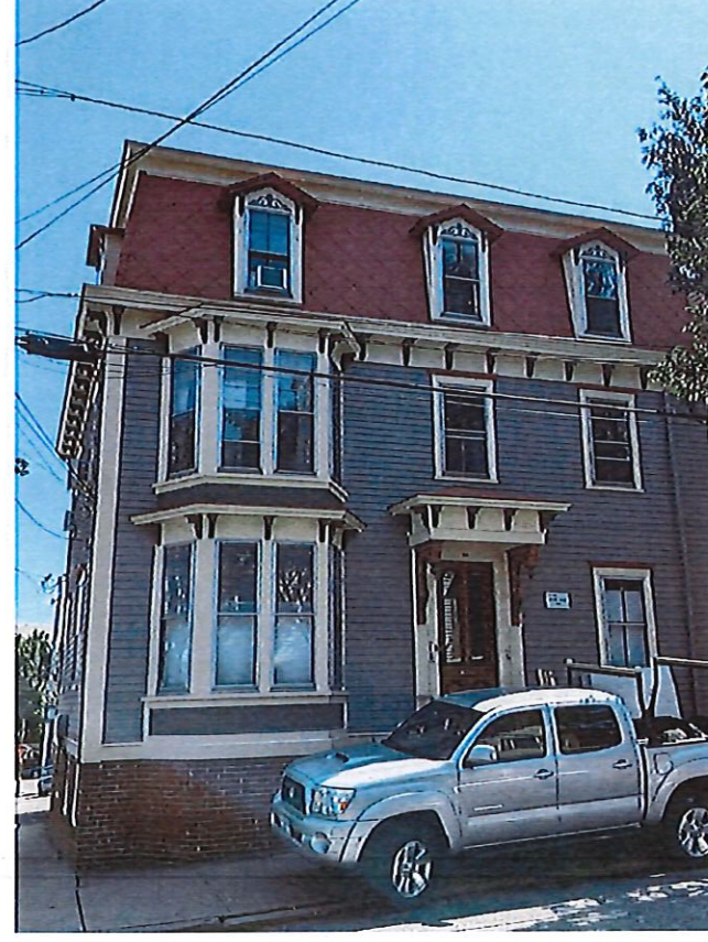
Existing View Sheldon Street
