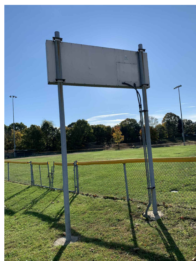
3 SOUTHERN FIELD SCOREBOARD 84.25" CENTER TO CENTER DISTANCE BETWEEN POLES
