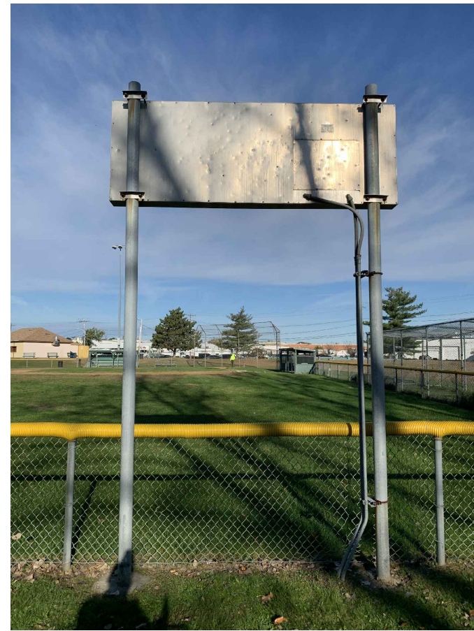
1 WESTERN FIELD SCOREBOARD 84.5" CENTER TO CENTER DISTANCE BETWEEN POLES
