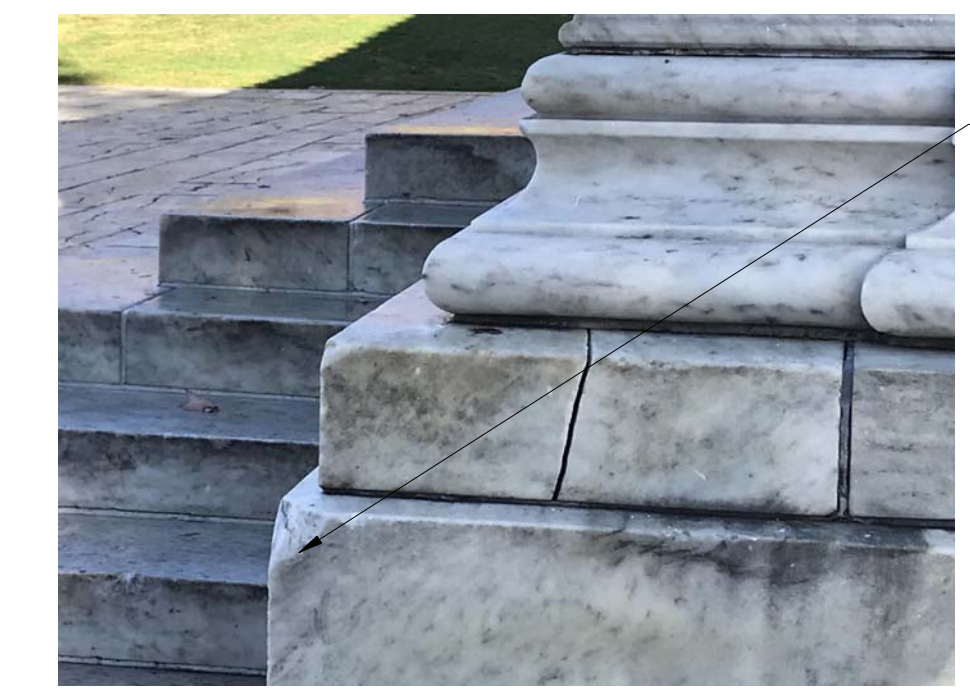
3 REPAIR CHIPPED STONE 1/16" = 1'-0"
