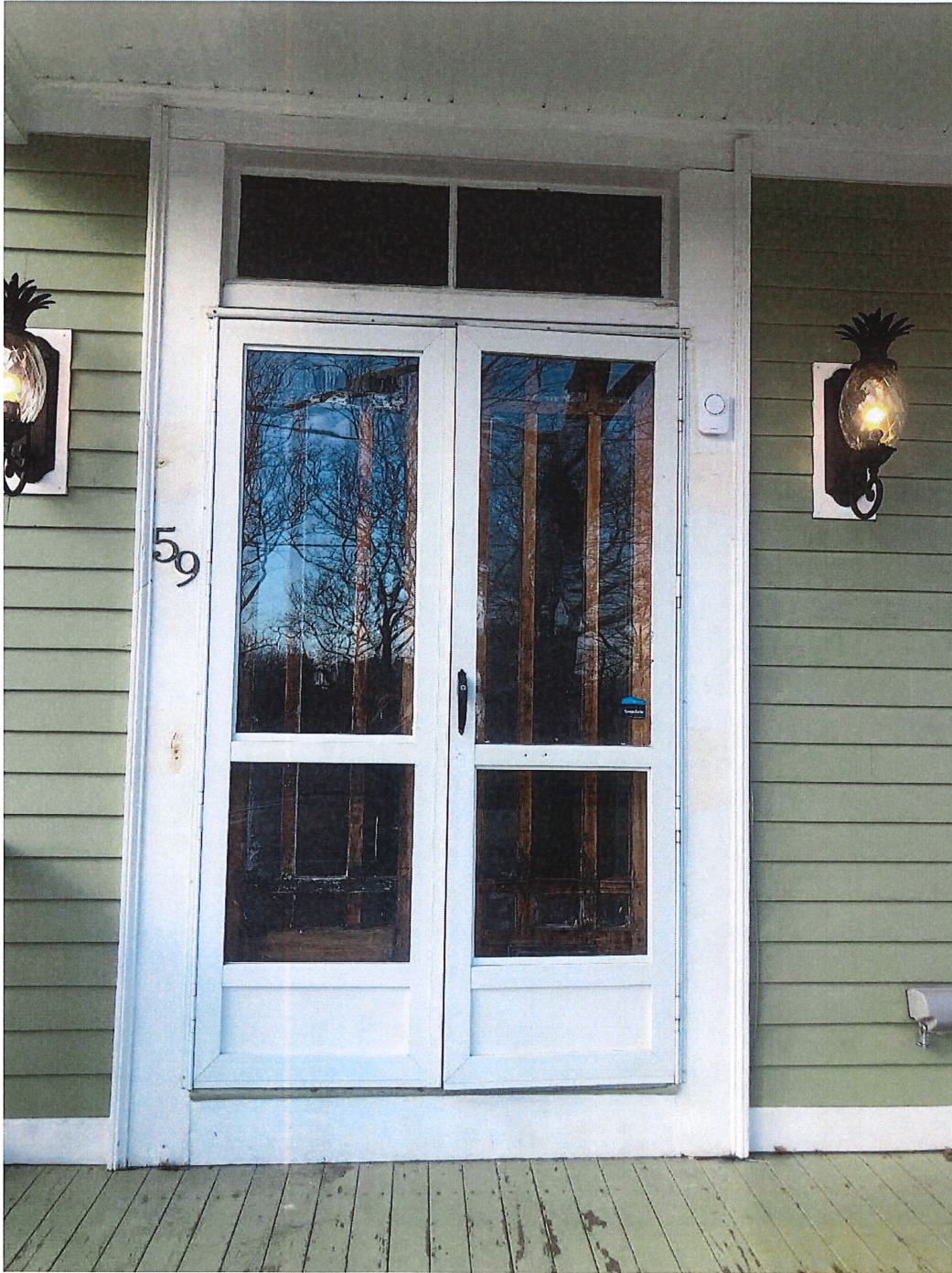
Figure 5 - Entry door to remain
