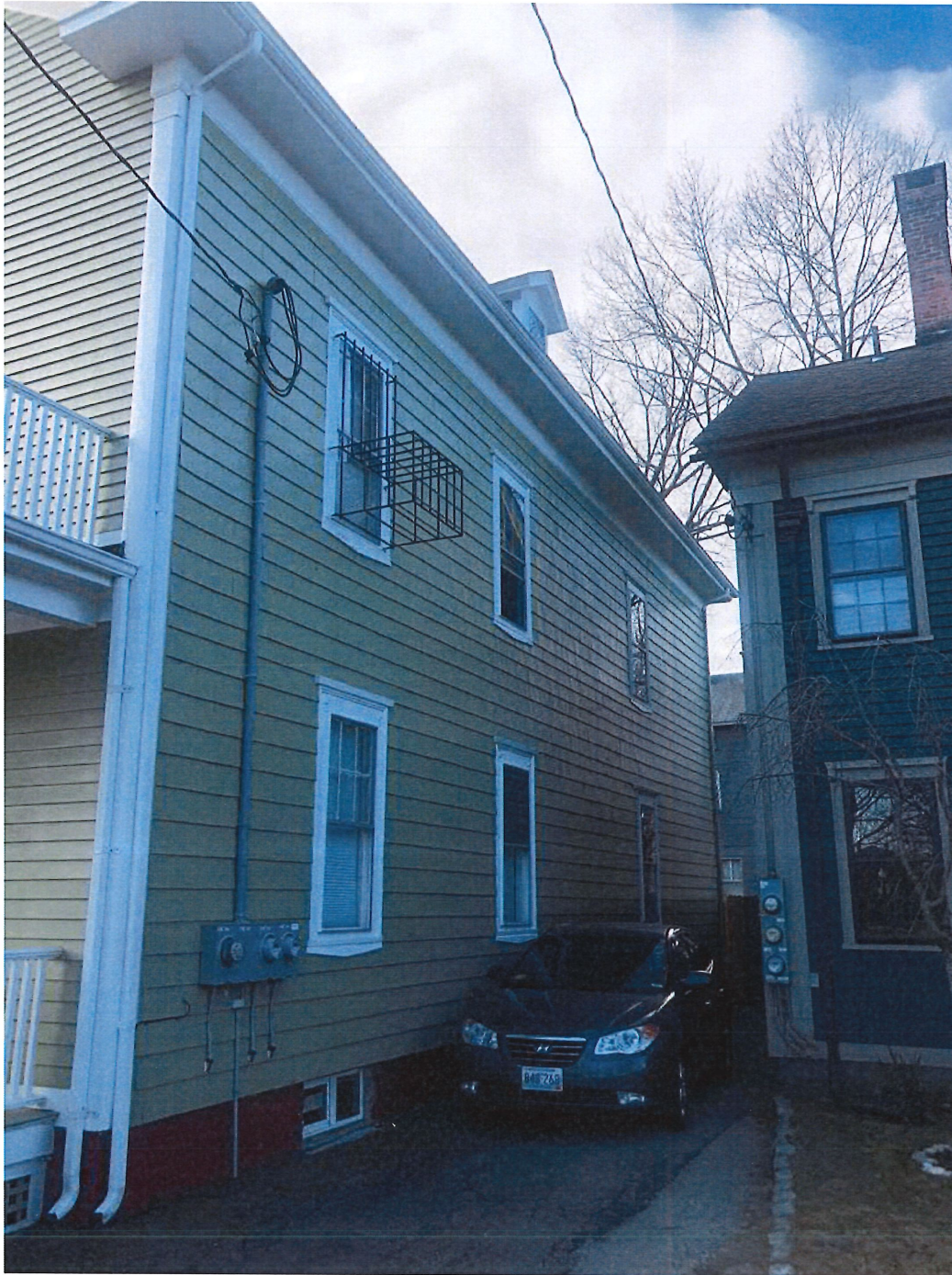
4- Side of building
