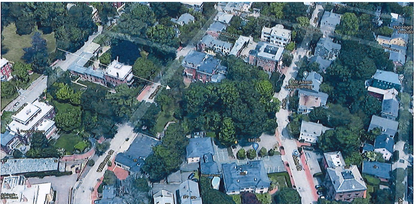
Arrow indicates project location, looking north.
