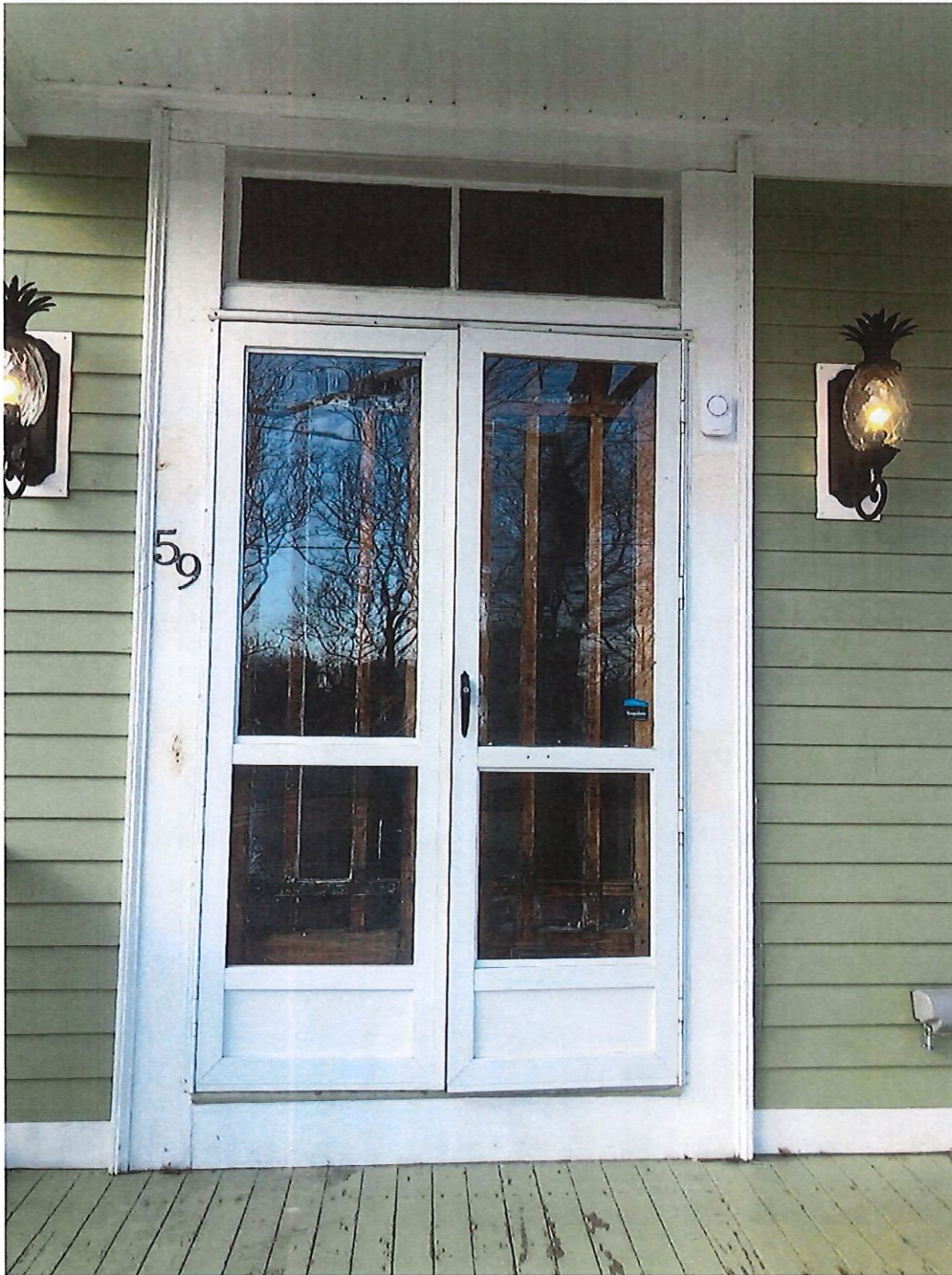
Figure 5 - Entry door to remain
