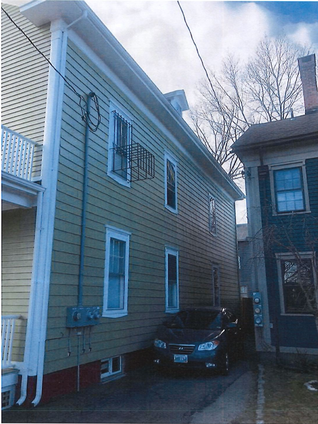
4- Side of building
