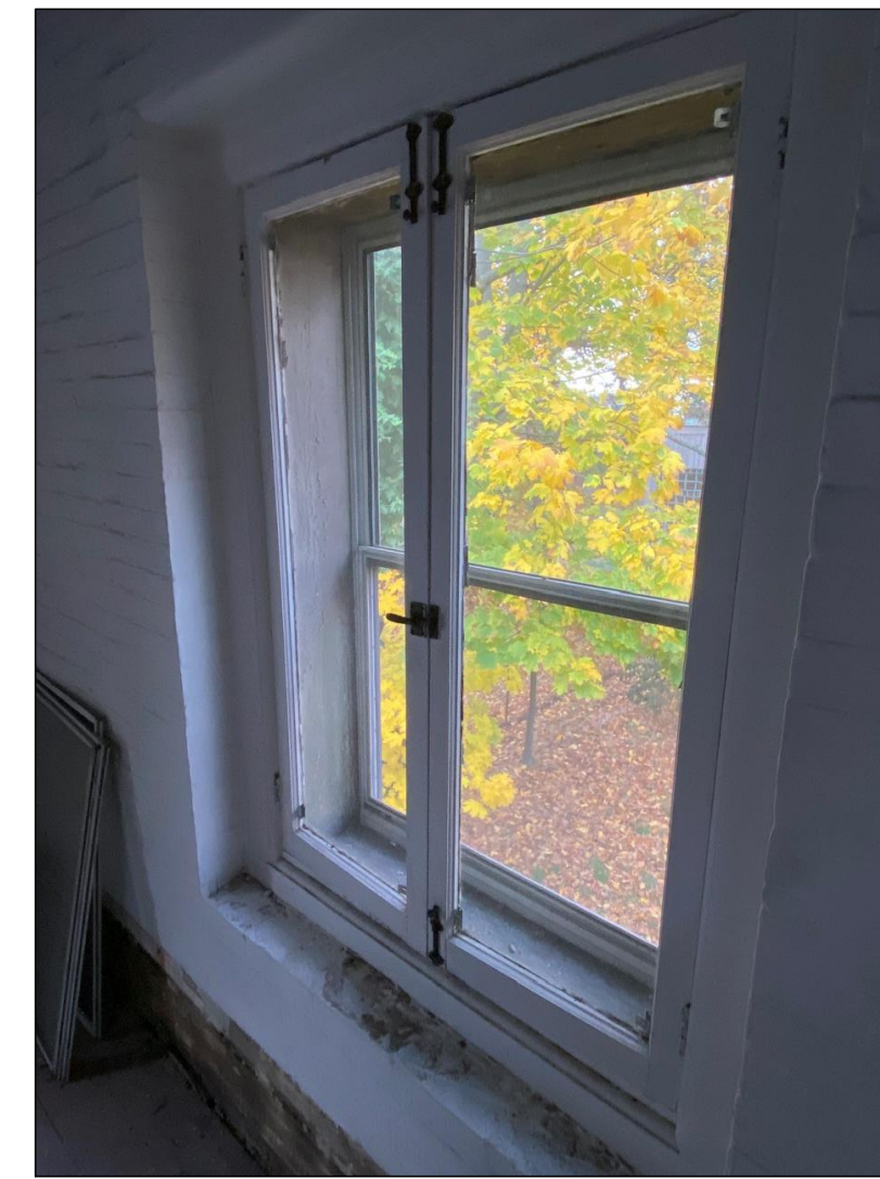
POSSIBLE ORIGINAL WOOD FRENCH CASEMENT WINDOWS (2ND FLOOR REAR)
