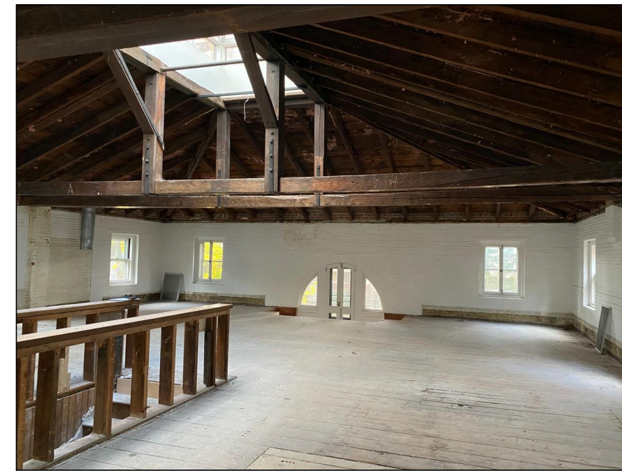
2ND FLOOR FROM NW CORNER LOOKING TOWARD REAR YARD (EXISTING CONDITIONS)
