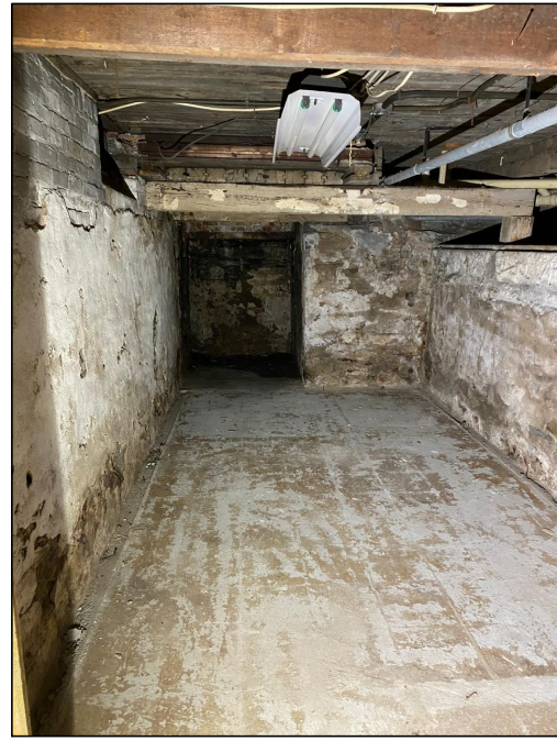
BASEMENT AREA UNDER PORTION OF FRONT ROOM
