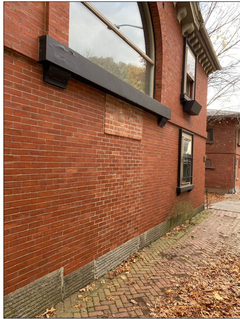
CLOSE UP OF MASONRY INFILL AT FORMER ENTRY DOOR
