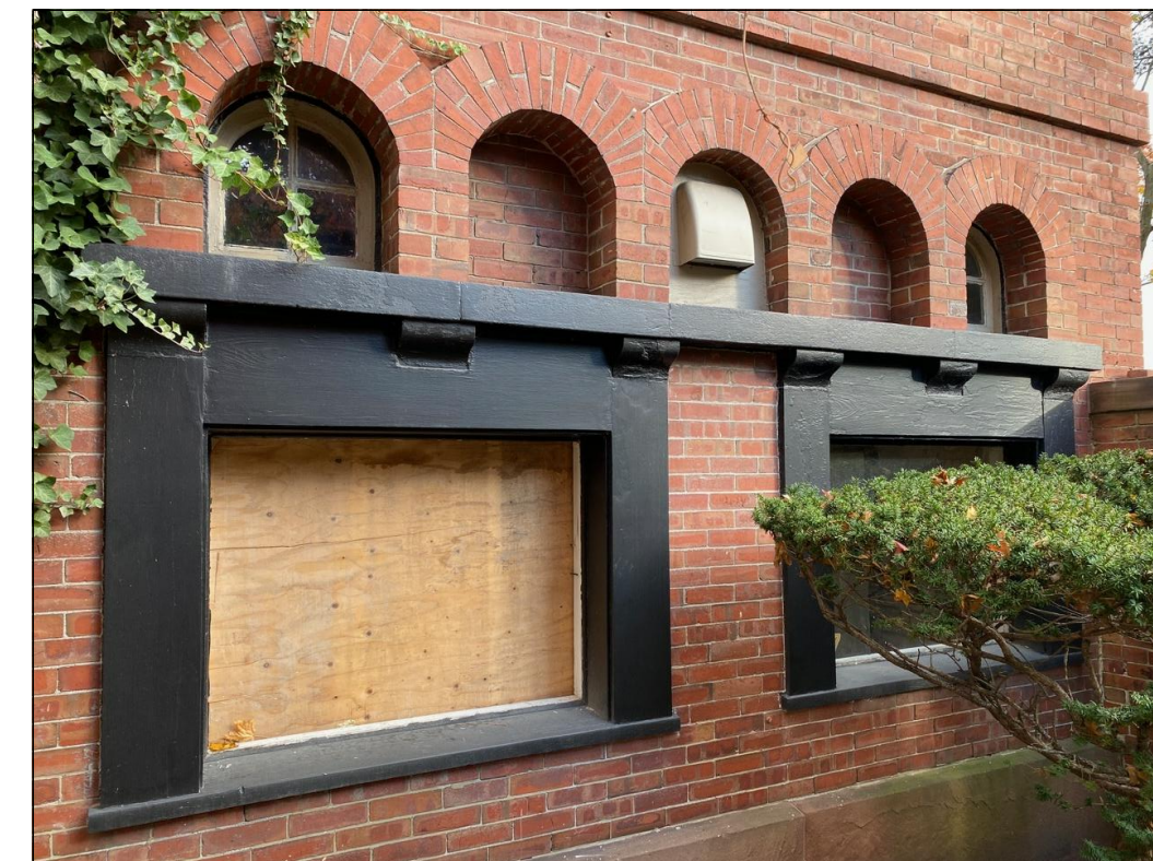
CLOSE UP VIEW OF NON-ORIGINAL WINDOWS BELOW ORIGINAL ARCHTOP CASEMENTS
