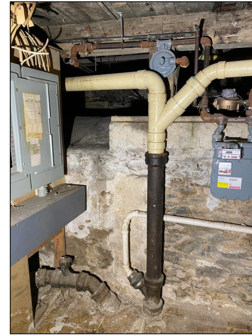
BASEMENT AREA UTILITIES
