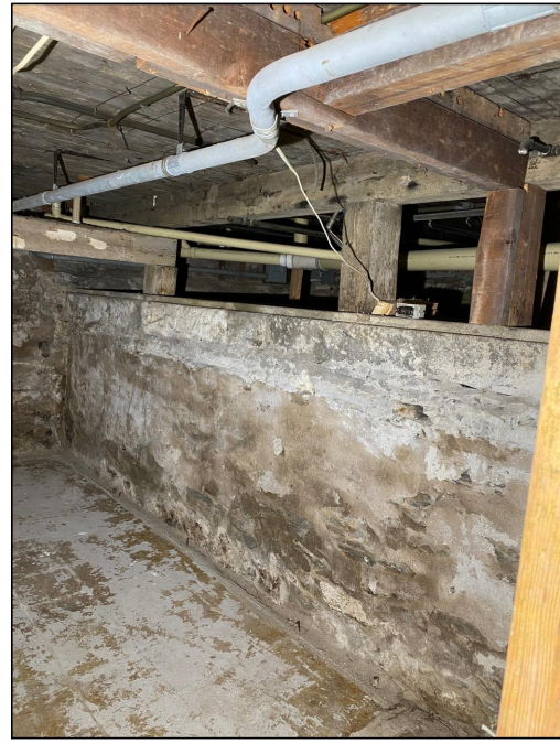
BASEMENT AREA LOOKING TO CRAWLSPACE UNDER REMAINDER OF FRONT ROOM
