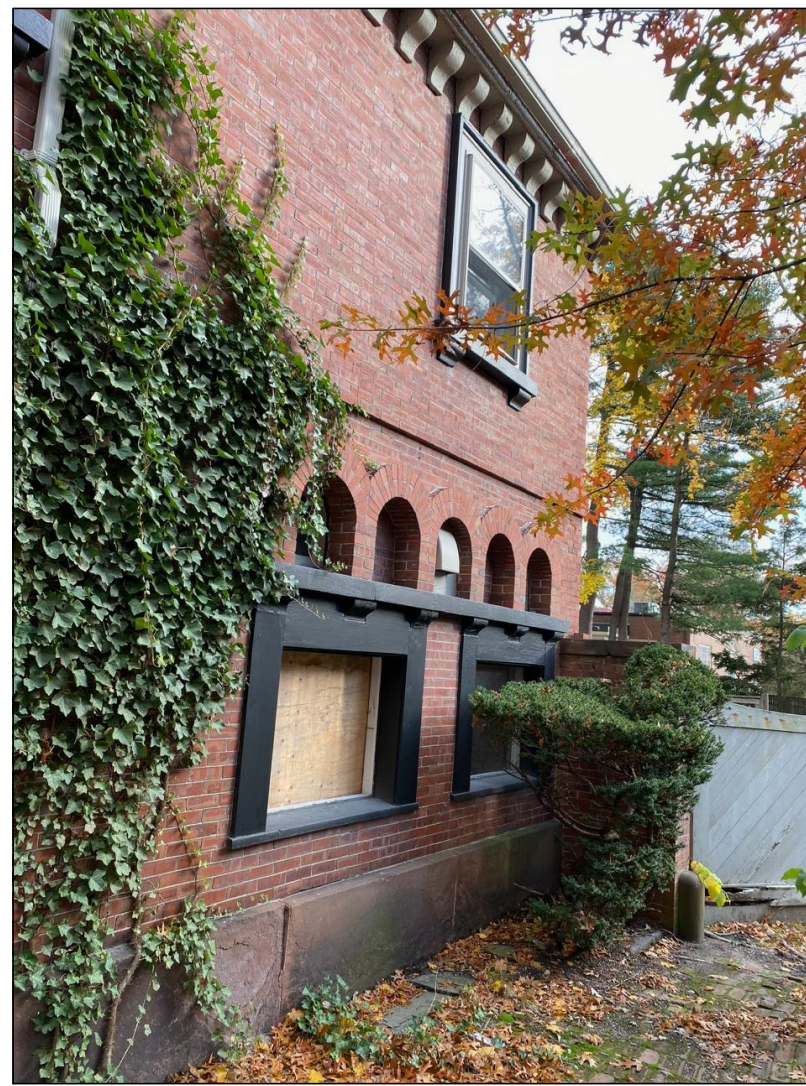
REAR HALF OF FACADE FROM CENTER OF DRIVEWAY
