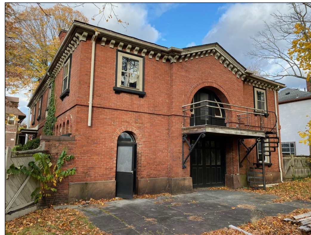
REAR FACADE FROM WEST SIDE OF REAR YARD
