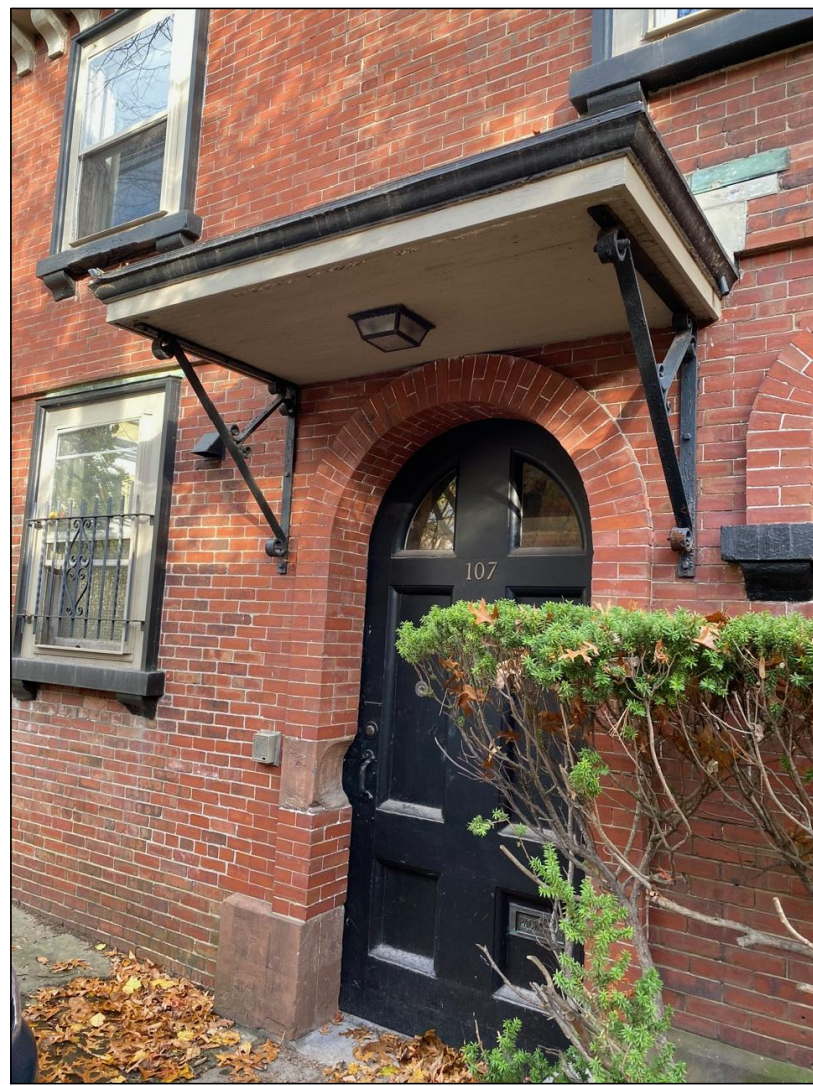
CLOSE UP VIEW OF CURRENT MAIN ENTRY DOOR
