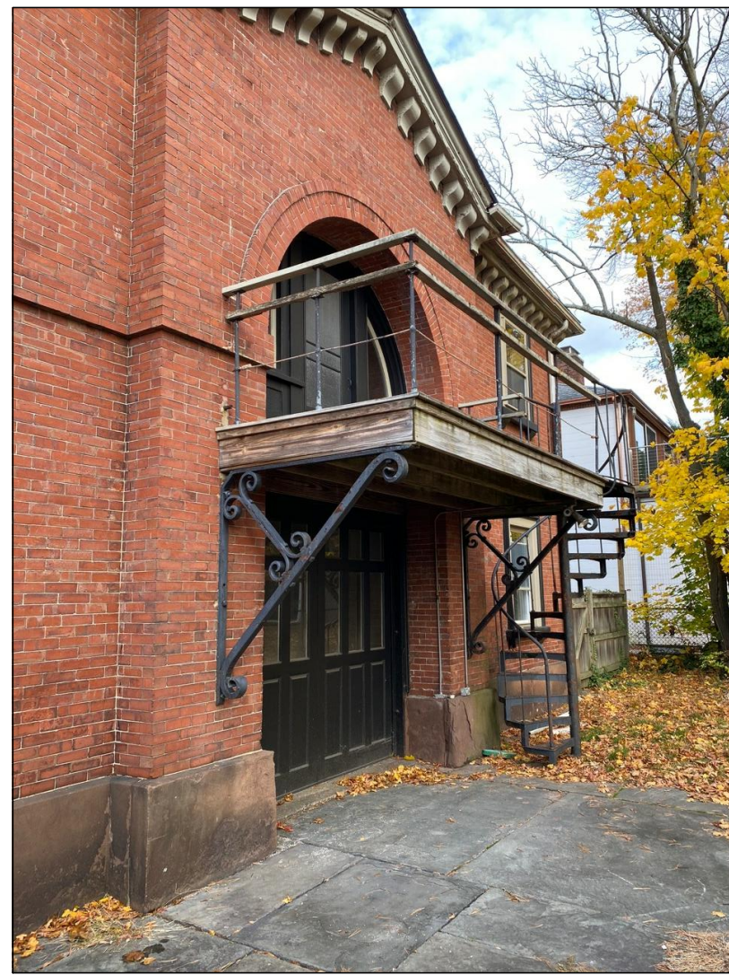
CLOSE UP VIEW ARCH TOP OPENING
