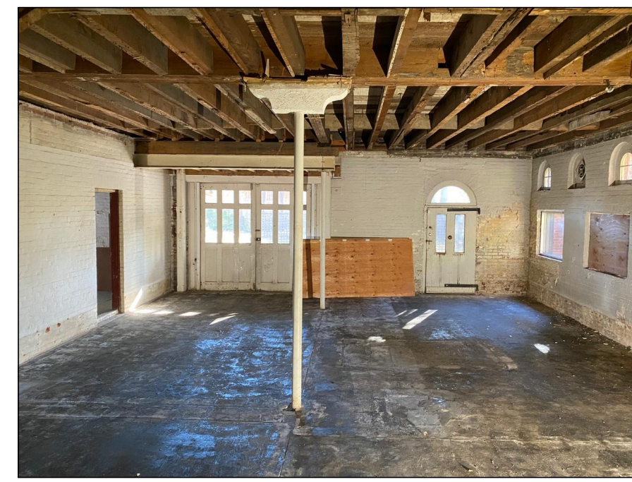
REAR SW ROOM LOOKING SOUTH TOWARD REAR YARD (EXISTING CONDITIONS)
