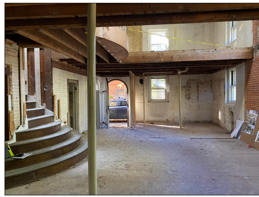
FRONT ROOM LOOKING WEST TOWARD DRIVEWAY (EXISTING CONDITIONS)
