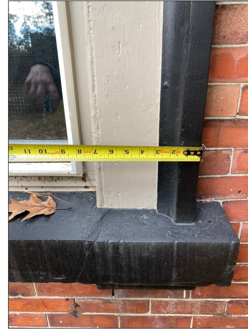
TYPICAL WINDOW CASING AND SILL CLOSEUP
