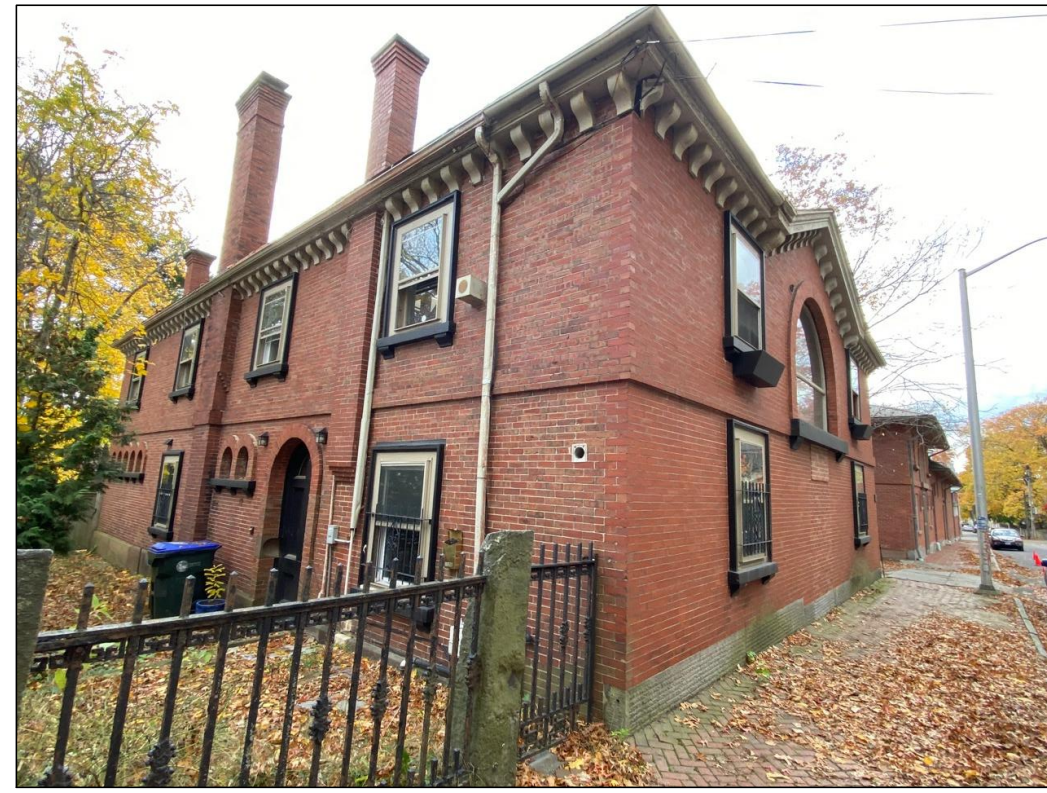
SIDE (EAST) AND FRONT (NORTH) FACADES FROM NEAR SIDEWALK ON BENEVOLENT STREET
