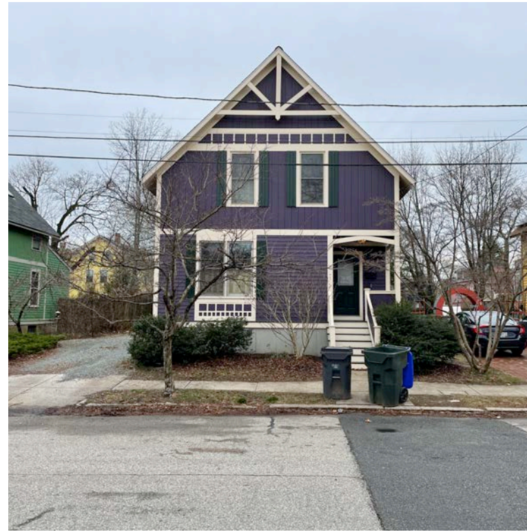
EXISTING PHOTOGRAPH: EAST (Note: this elevation not affected by proposed changes)
