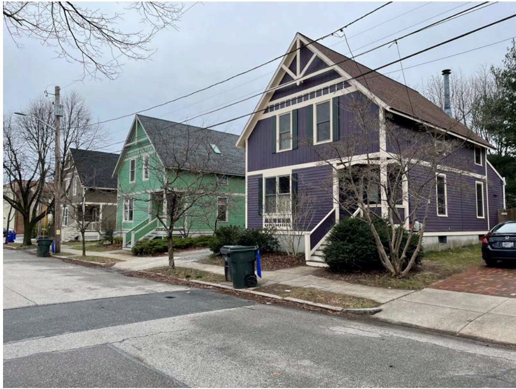
EXISTING PHOTOGRAPH: VIEW FROM NORTHEAST (HAMMOND STREET)
