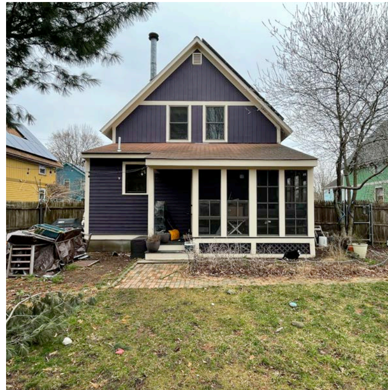
EXISTING PHOTOGRAPH: WEST
