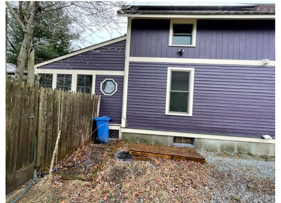
EXISTING PHOTOGRAPH: PARTIAL SOUTH ELEVATION
