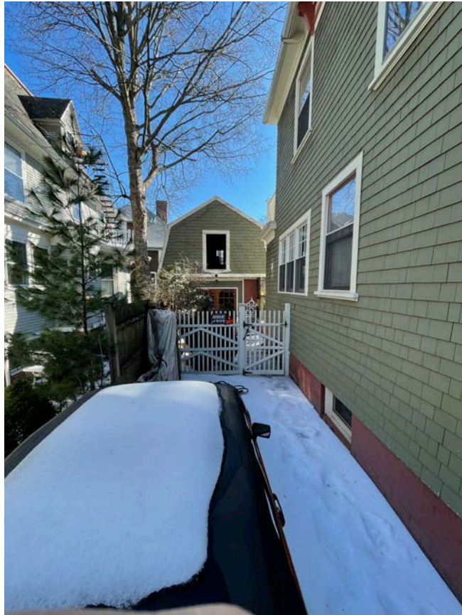
VIEW FROM WEST (GOVERNOR STREET)
