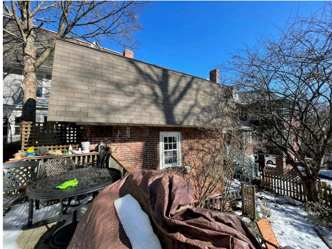
VIEW FROM BACK DECK (SOUTHWEST)
