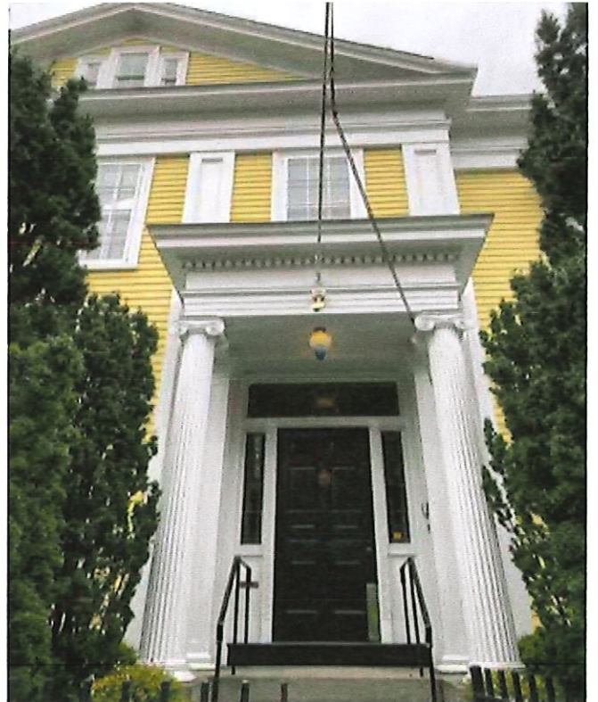
NORTH ENTRANCE ELEVATION
