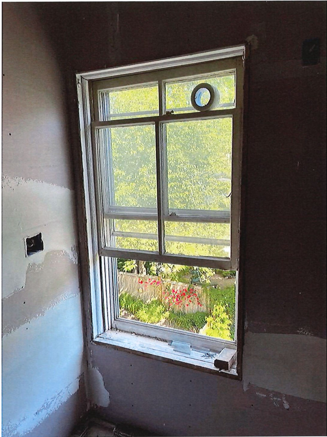
Figure 6 - Interior of 2/2, type "B" unit
