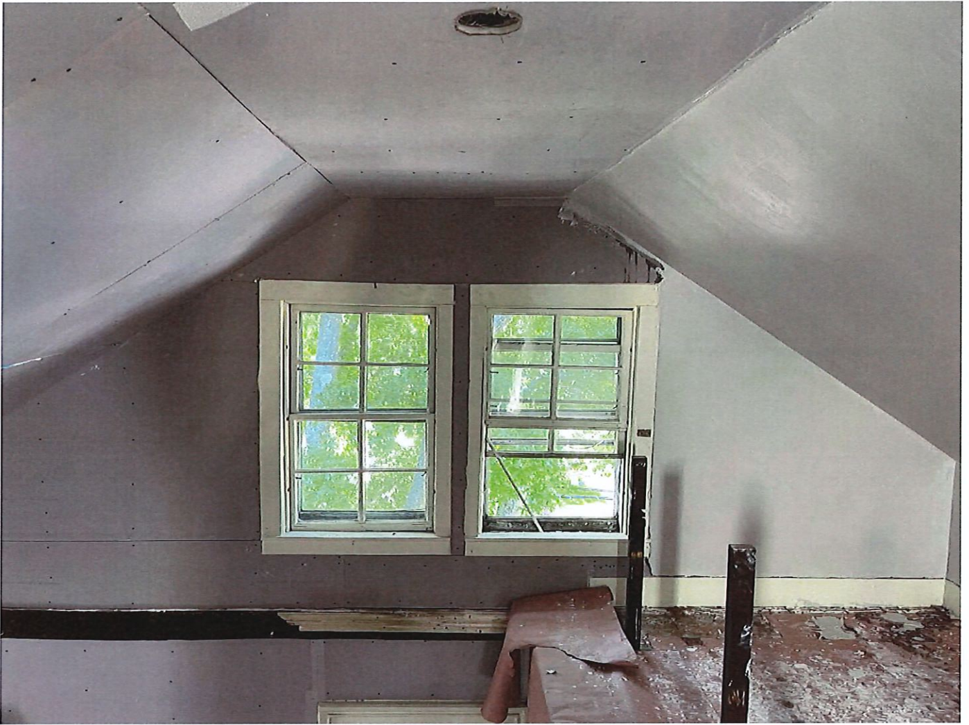
Figure 7 - interior of 4/4, type "C" unit at loft level
