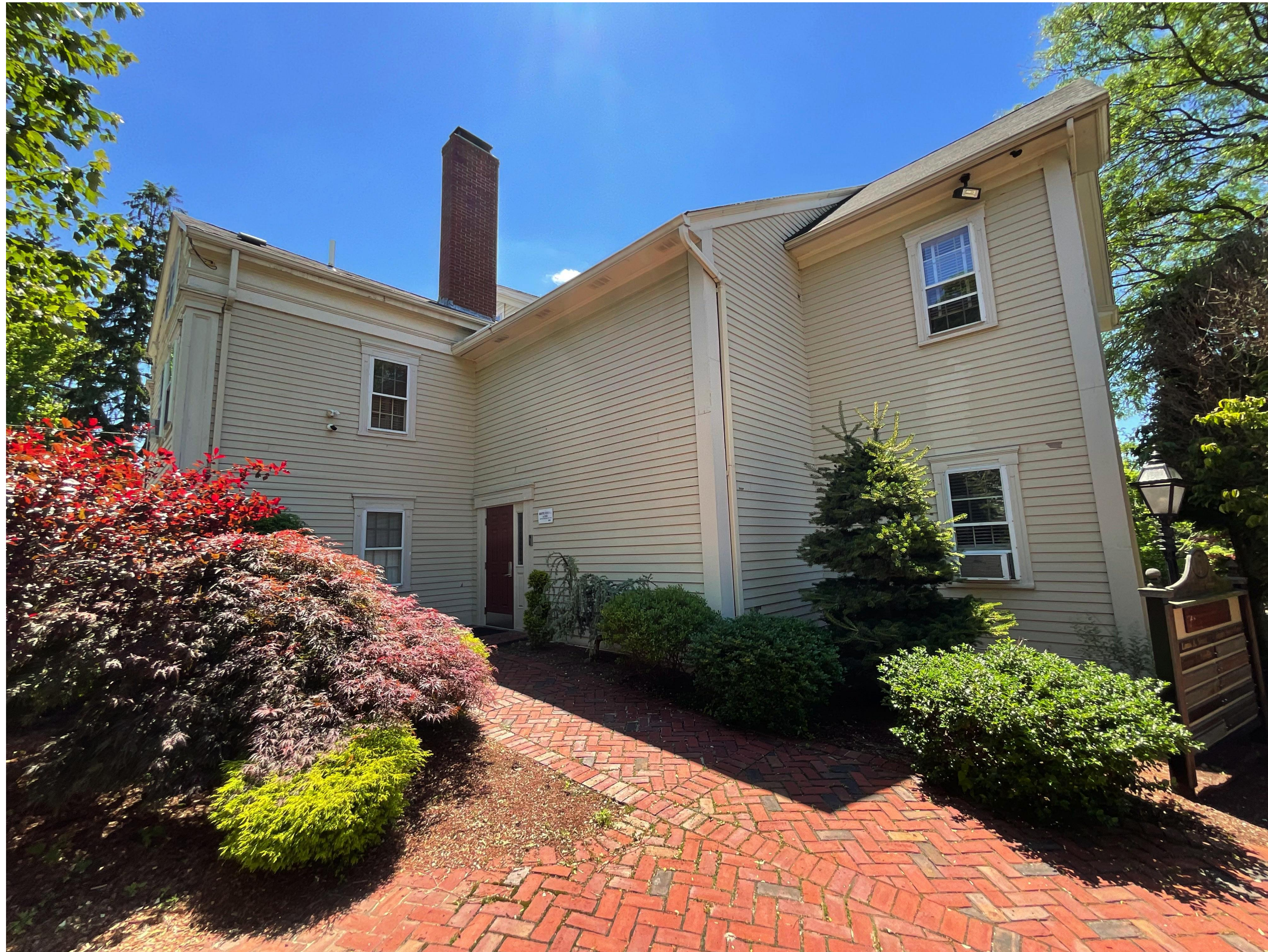
EXISTING NORTH EAST CORNER OF BUILDING AT LOCATION OF PROPOSED EXTERIOR STAIRCASE
