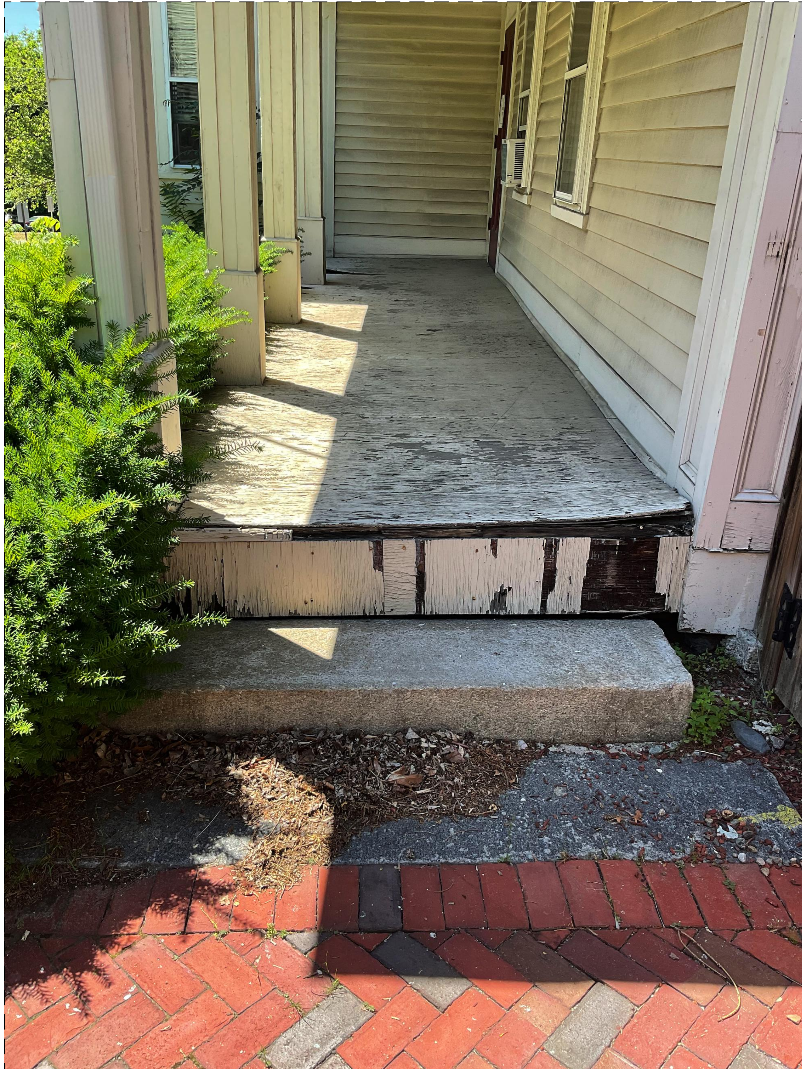
Existing Side Porch Conditions
