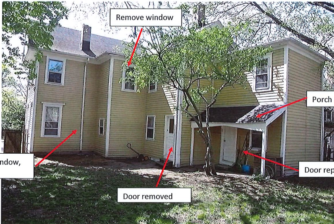
Figure 4 - View from SE corner prior to work
