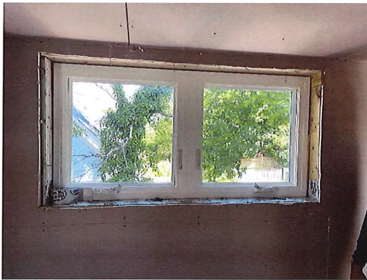
Figure 14 - unit "M" from interior
