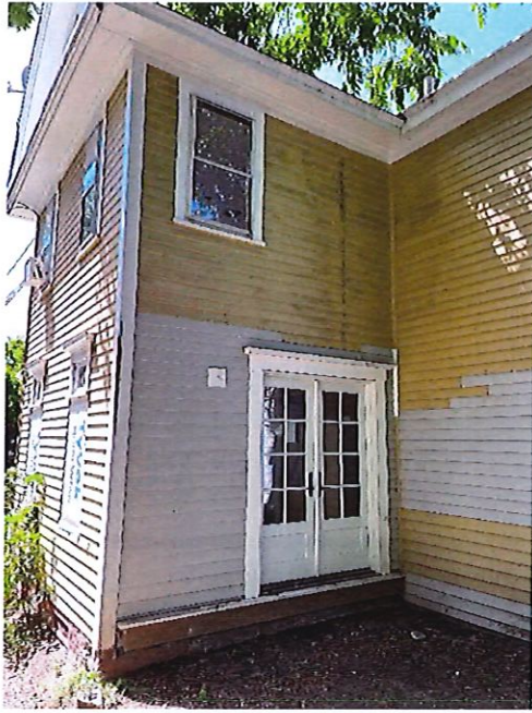
Figure 5 - View of ne door on east
