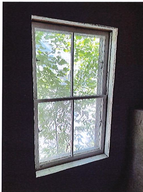
Figure 12 - existing DH unit to be replaced
