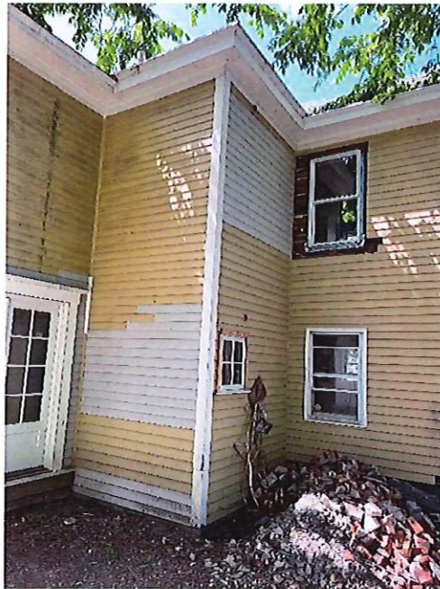
Figure 6 - new and infilled units
