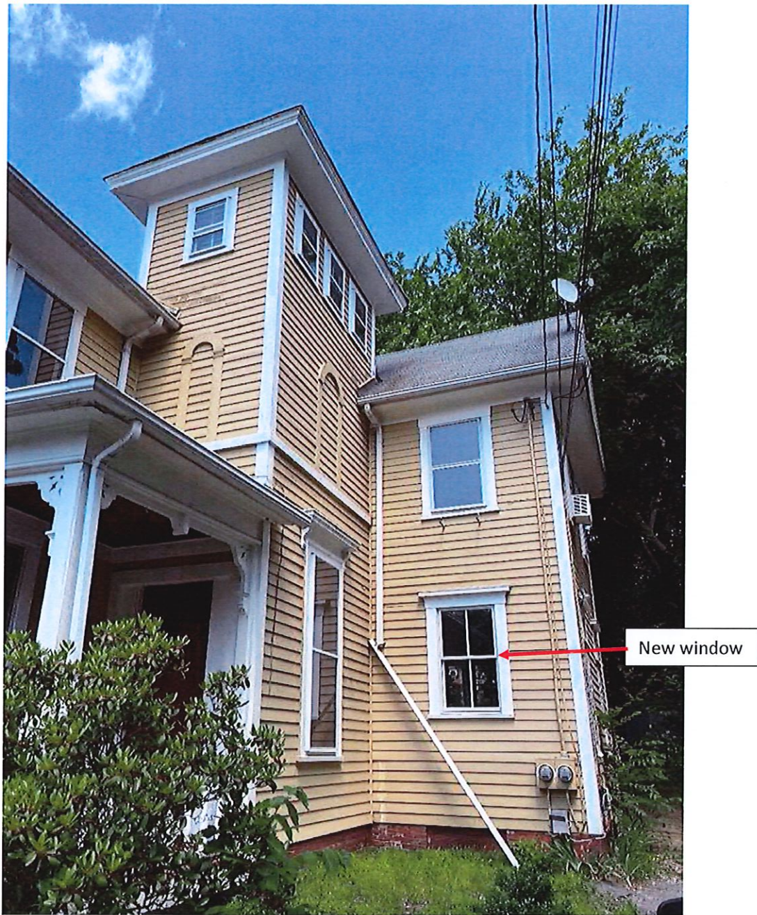
Figure 2 - View of tower
