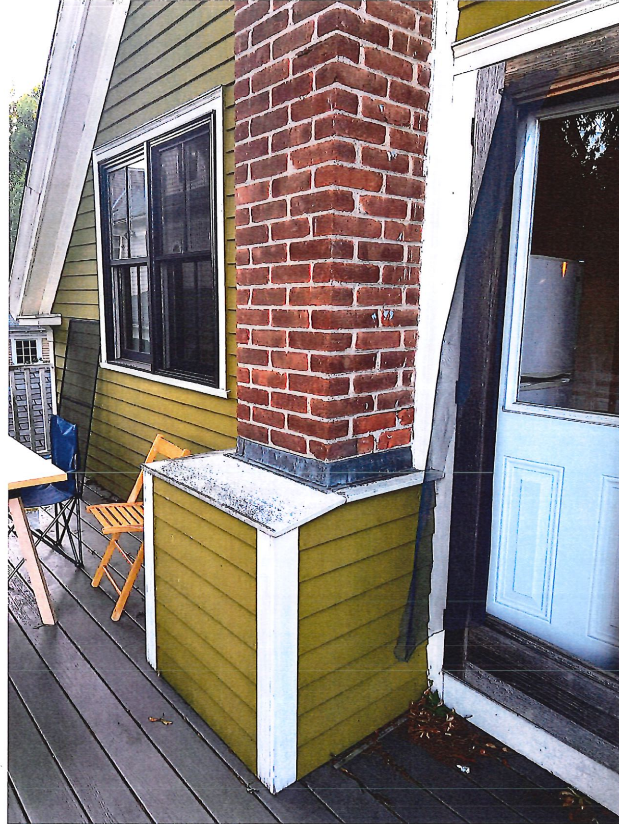
Photo: Chimney Base on Porch
