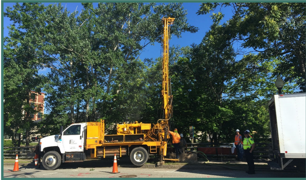
Soil Boring being completed at the Project site, photo taken by RTG on June 17, 2019.
