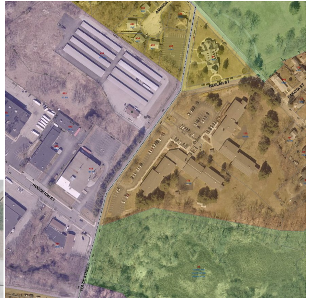
An aerial view of the site
