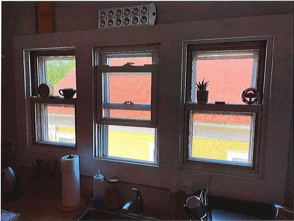
Figure 13 - Triple DH units to be changed to pair of Awning
