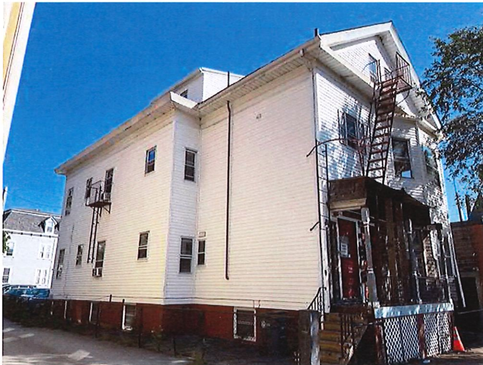
Figure 5 - west side and entry porch
