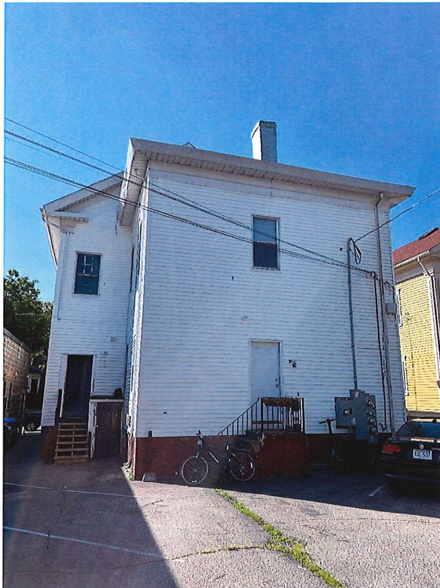
Figure 3 - North (rear) side
