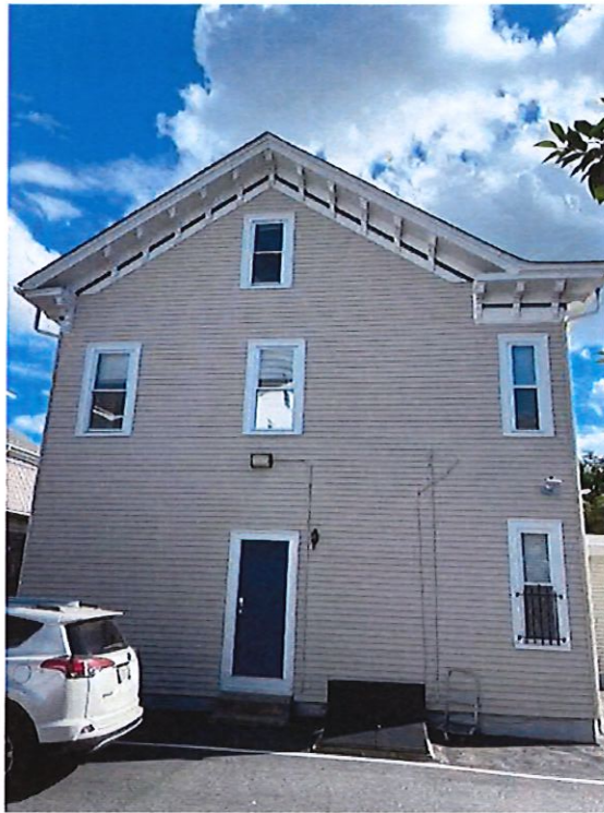
Figure 5 - View from rear (north) window "B"
