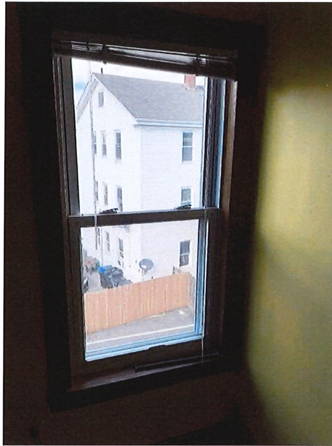
Figure 7 - detail window "B"
