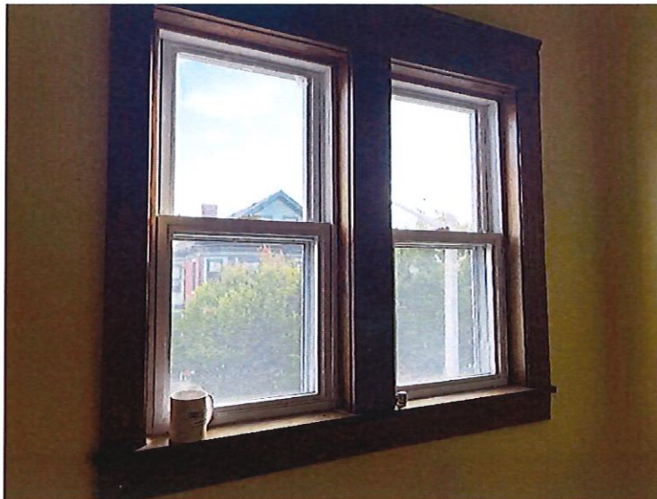
Figure 3 - Interior at window "A"
