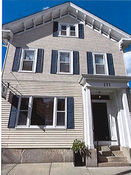
Figure 1 - View from Broadway (south) window "A"
