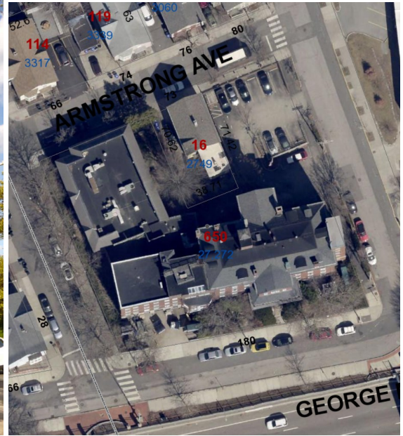
Aerial view of the site
