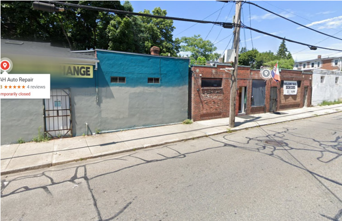
View of the building from Douglas Ave
