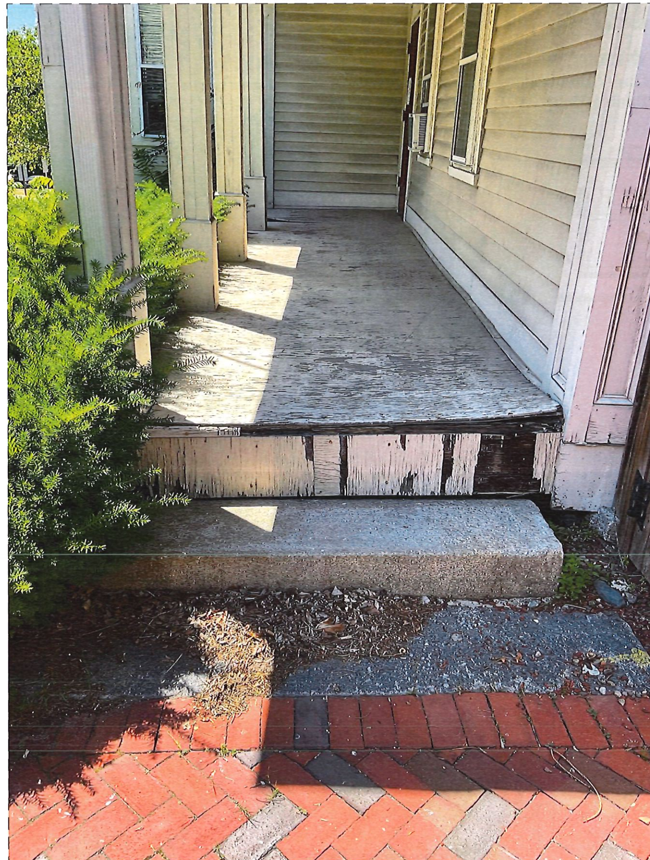
Existing Side Porch Conditions
