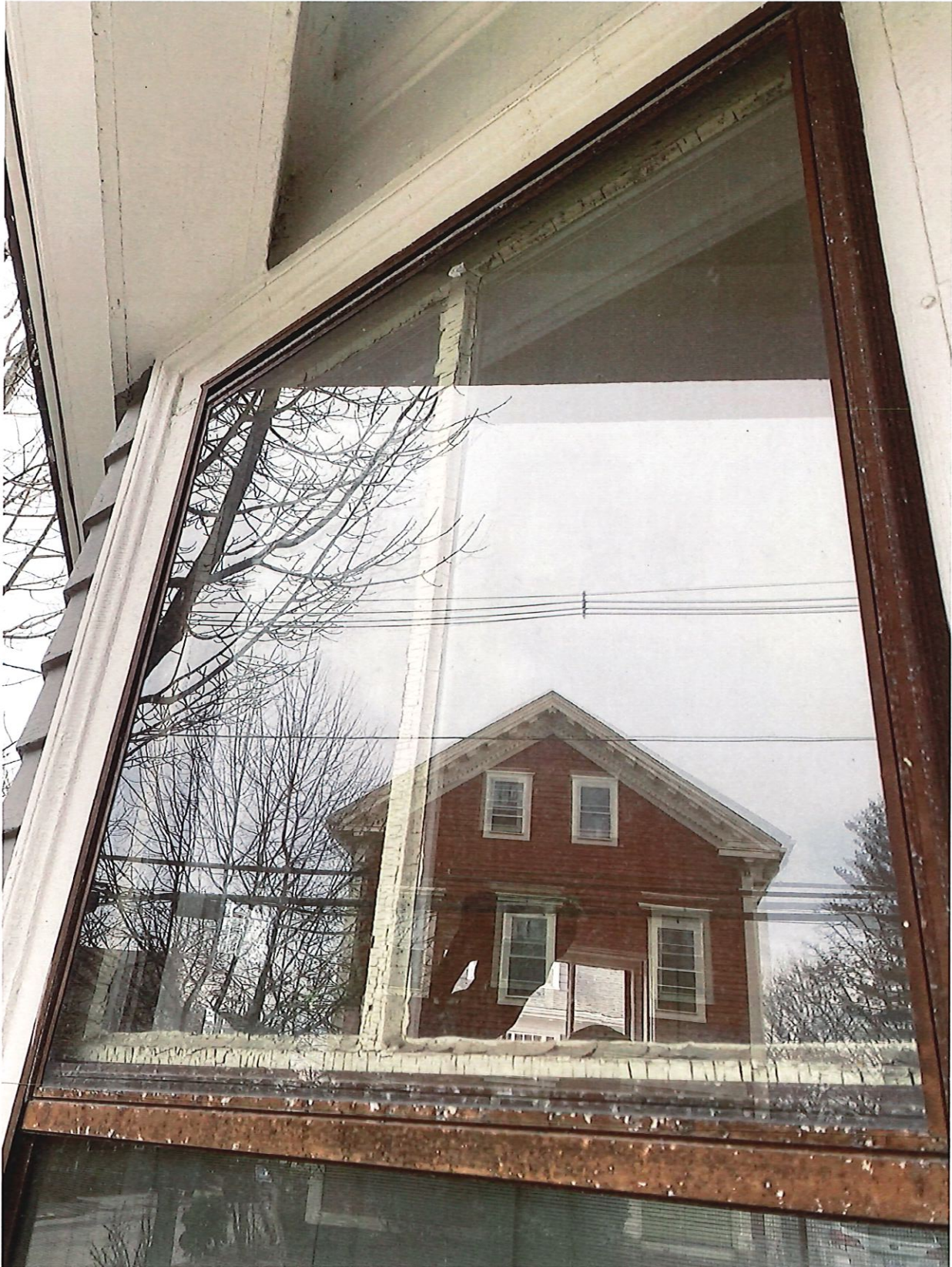
Condition of Original Windows
