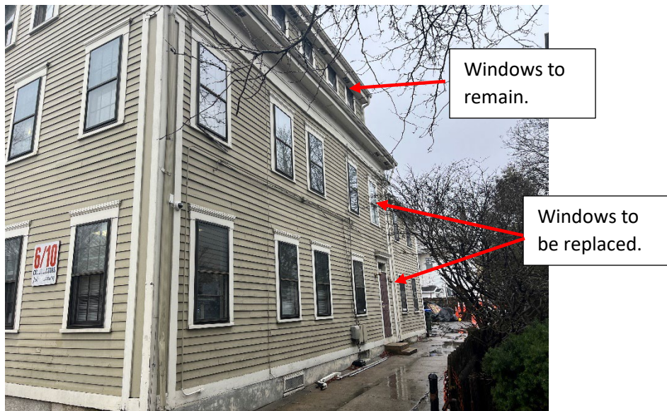
Figure 2 - Side view west
