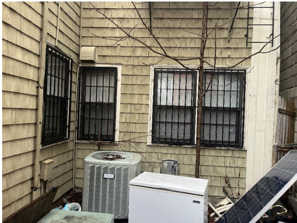
Figure 4 - detail view from south
