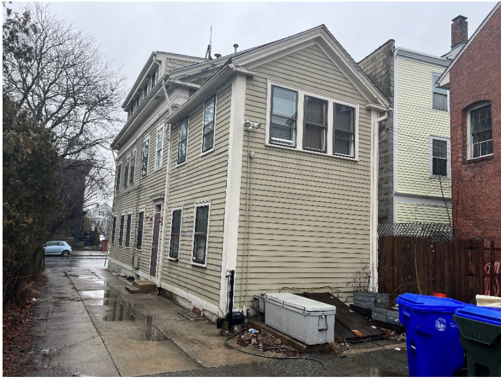
Figure 3 - view from back (south)
