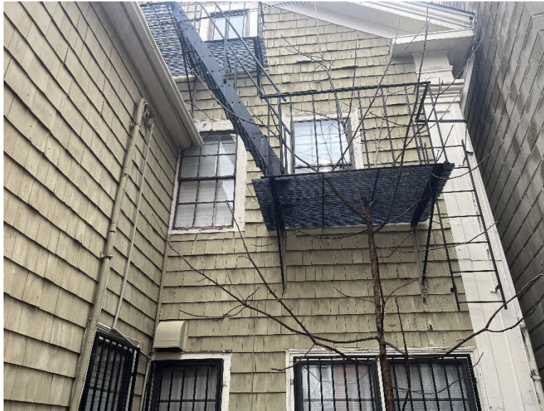
Figure 5 - detail view from south
