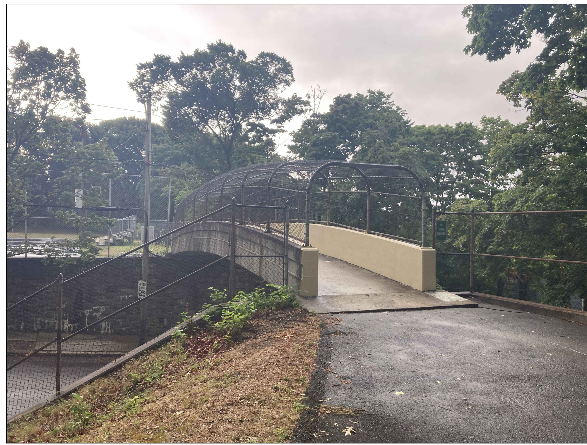
BILLY TAYLOR OVERPASS OPPOSITE SIDE OF CYPRESS STREET
