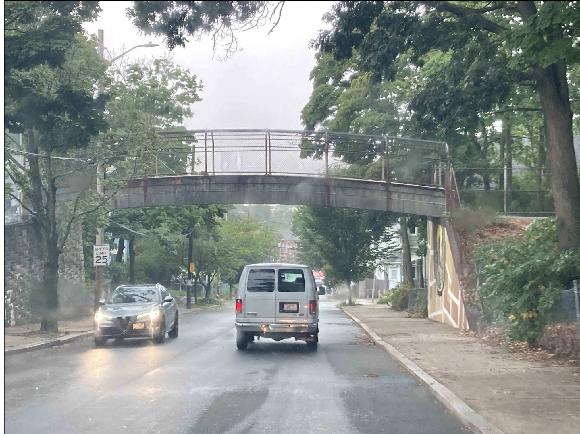
BILLY TAYLOR OVERPASS VIEW FROM CYPRESS ST.
