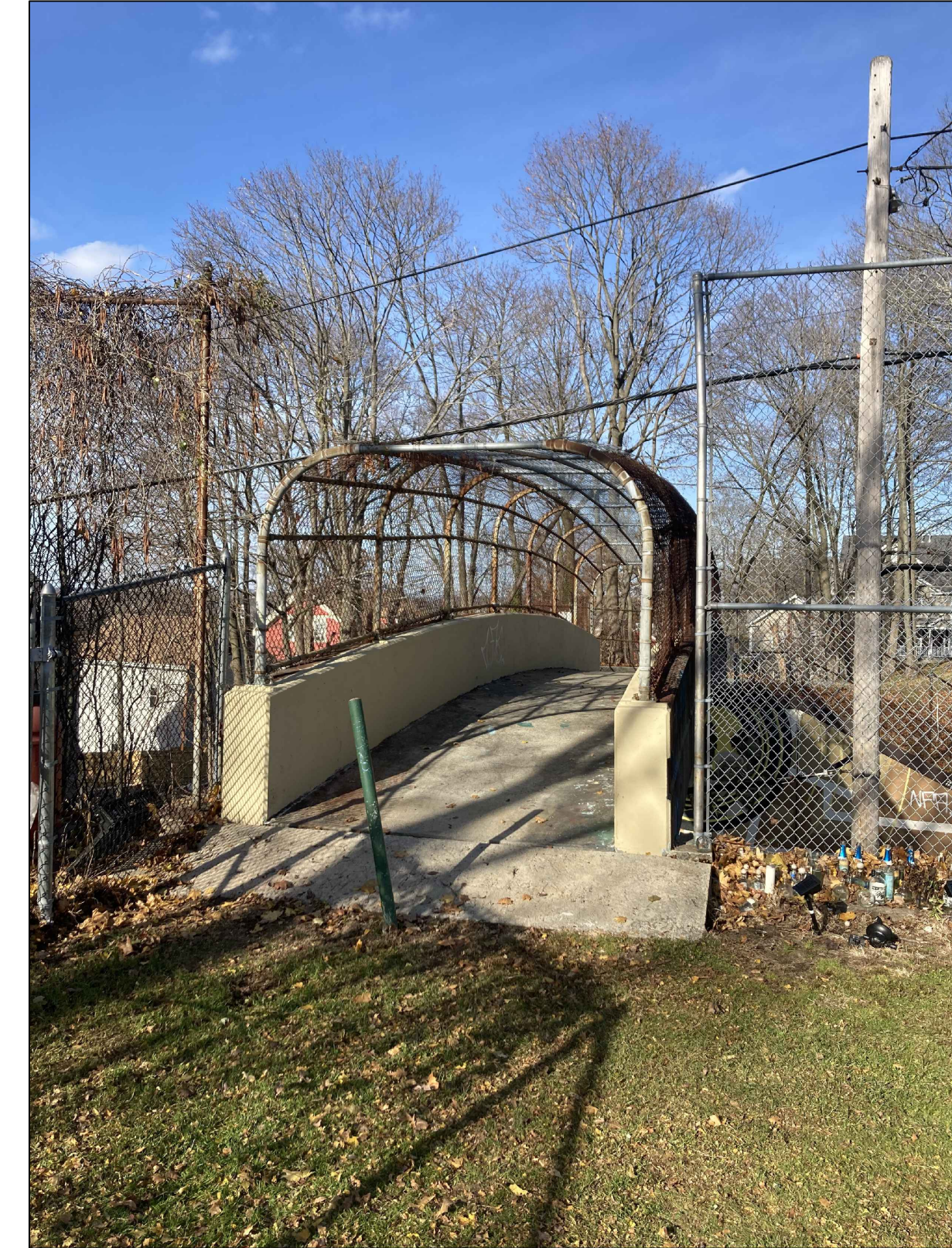
BILLY TAYLOR OVERPASS APPROACH - PARK SIDE
