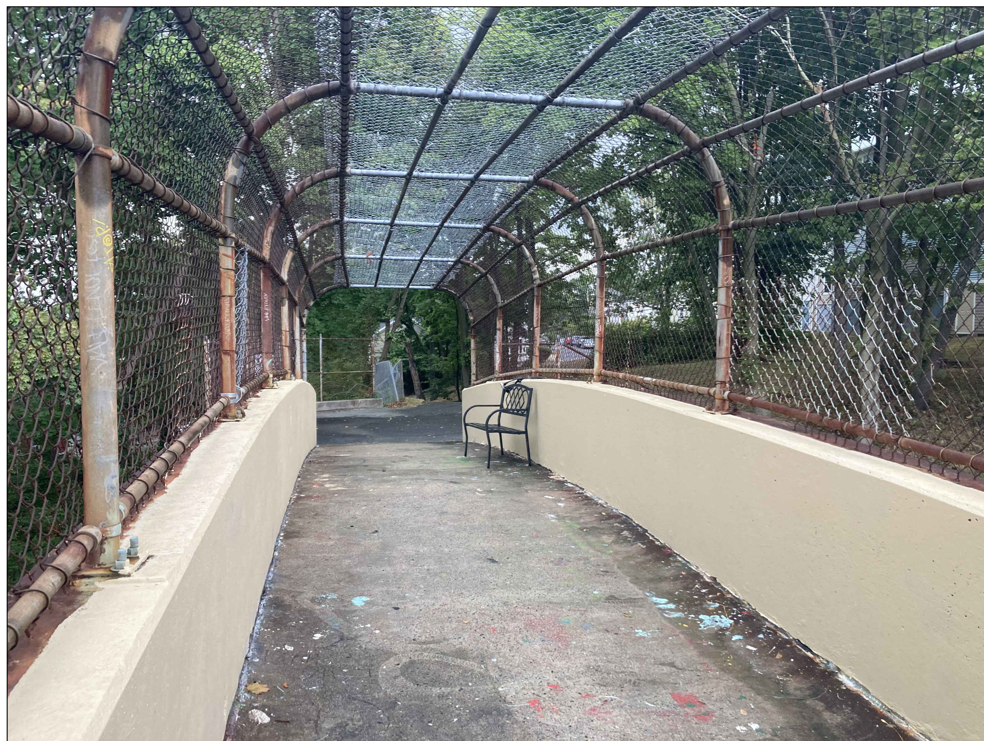
BILLY TAYLOR OVERPASS INTERIOR VIEW
