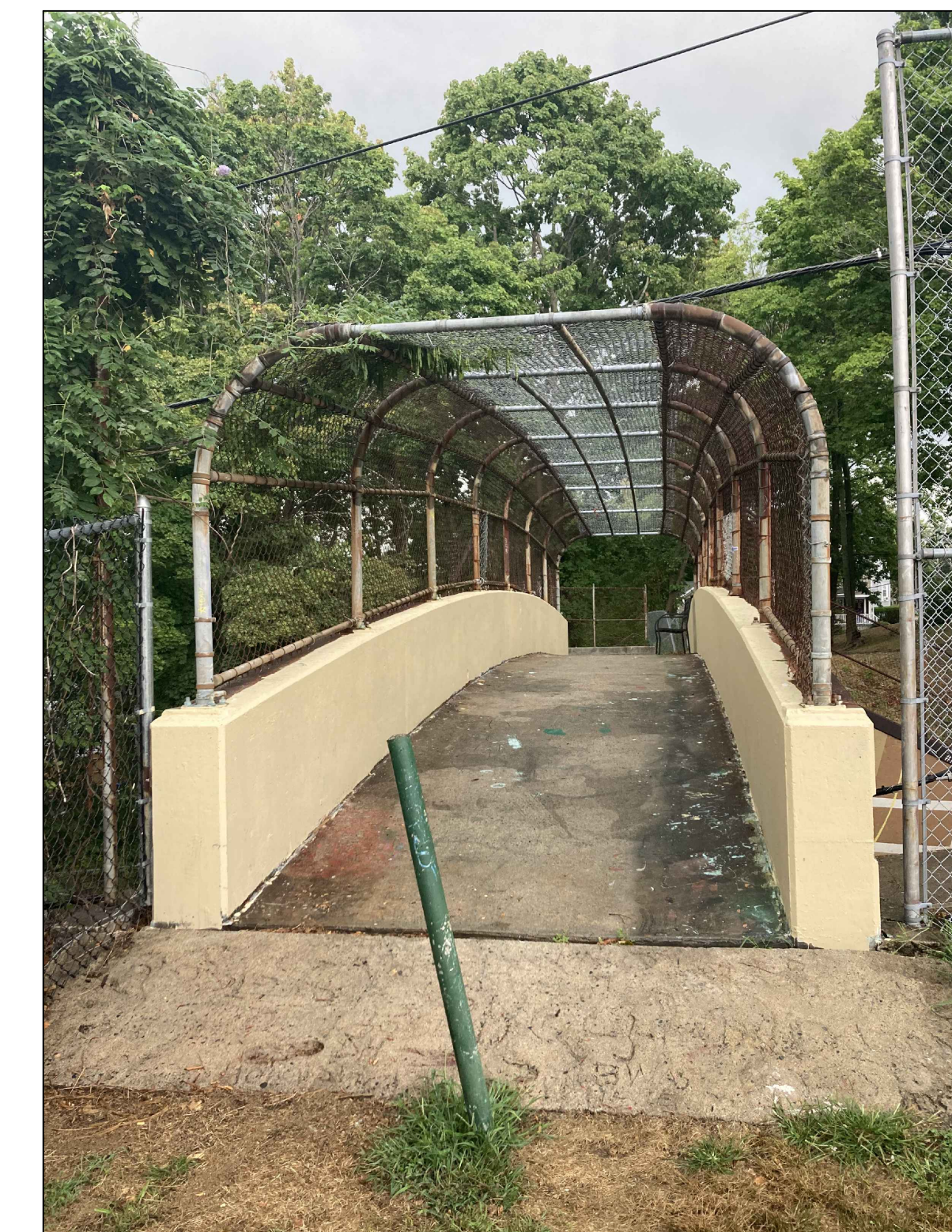
BILLY TAYLOR OVERPASS INTERIOR VIEW
