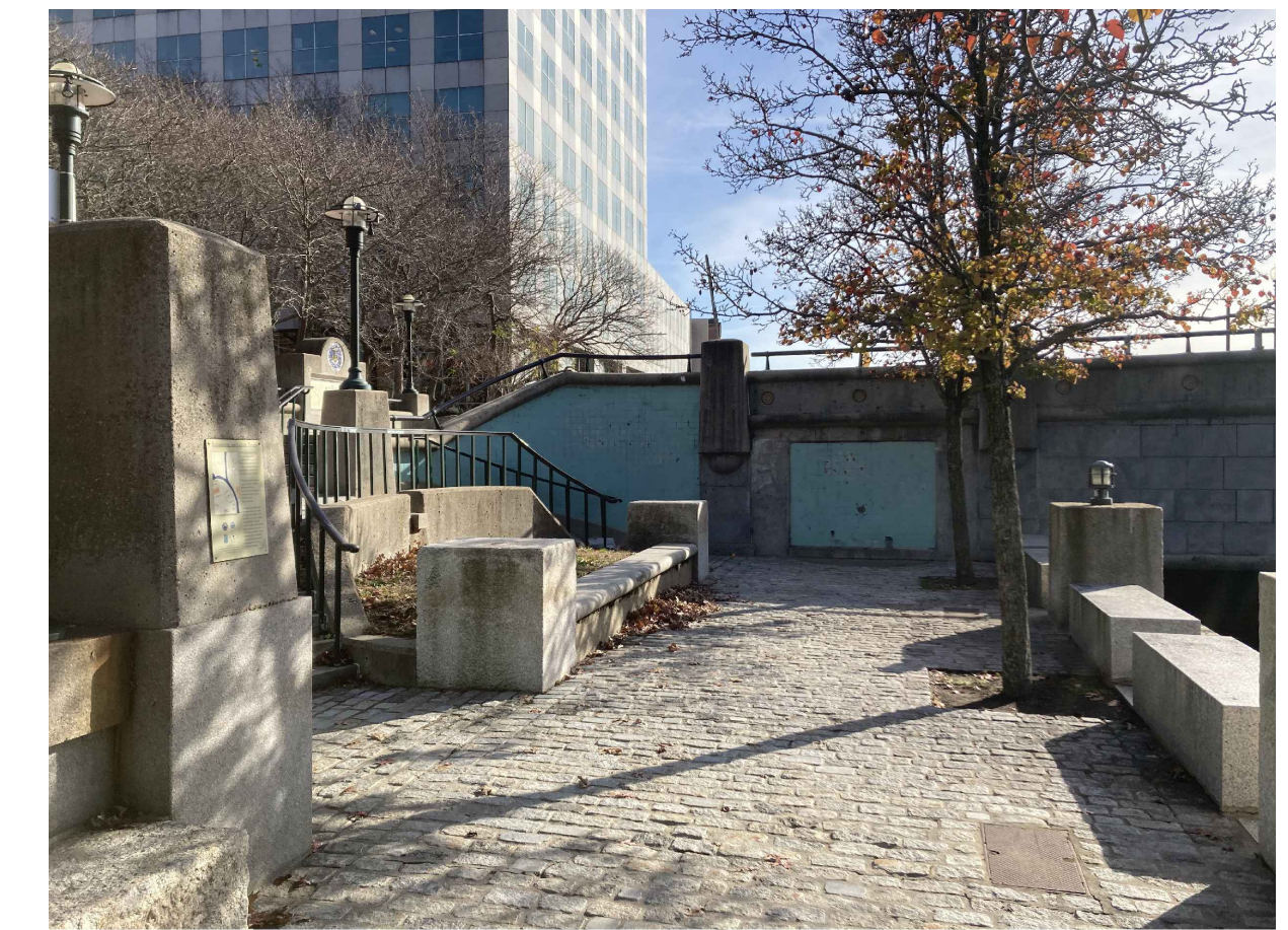
VIEW OF TILED PANELS 'B' & 'C' TOWARDS CRAWFORD STREET BRIDGE
