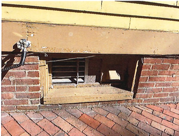
Figure 8 - Unit "D" at basement
