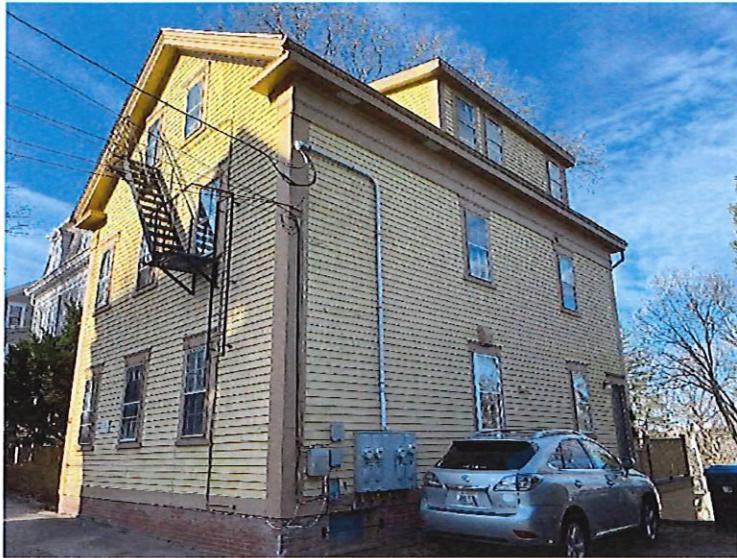
Figure 3 - view from NE
