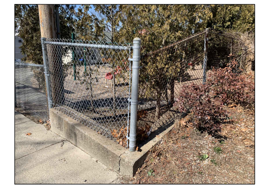
6 VIEW FROM PLEASANT ST AT NORTHEAST CORNER
