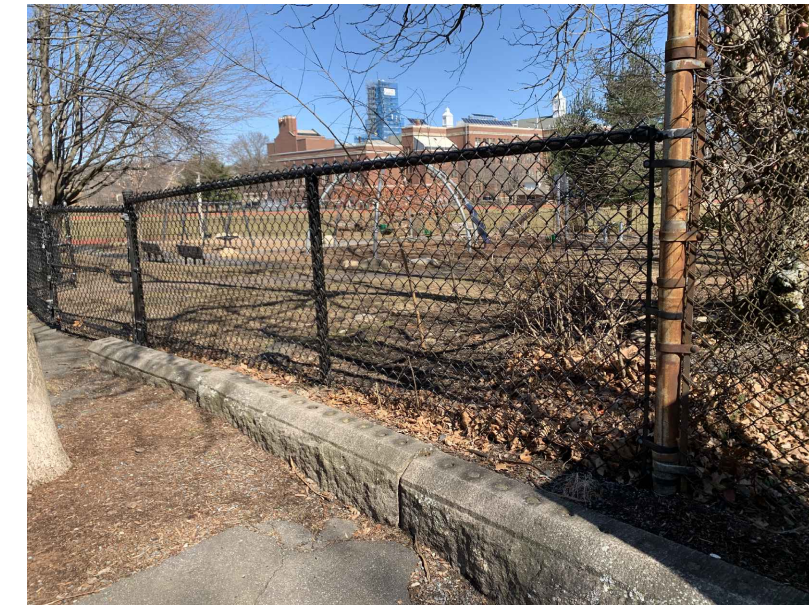
6 VIEW FROM BROWN ST AT SOUTH FENCE CORNER
