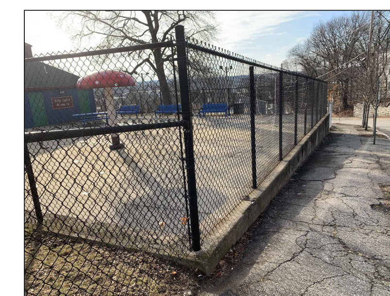
6 VIEW OF EXISTING CL FENCE TO REMAIN ON CYPRESS
