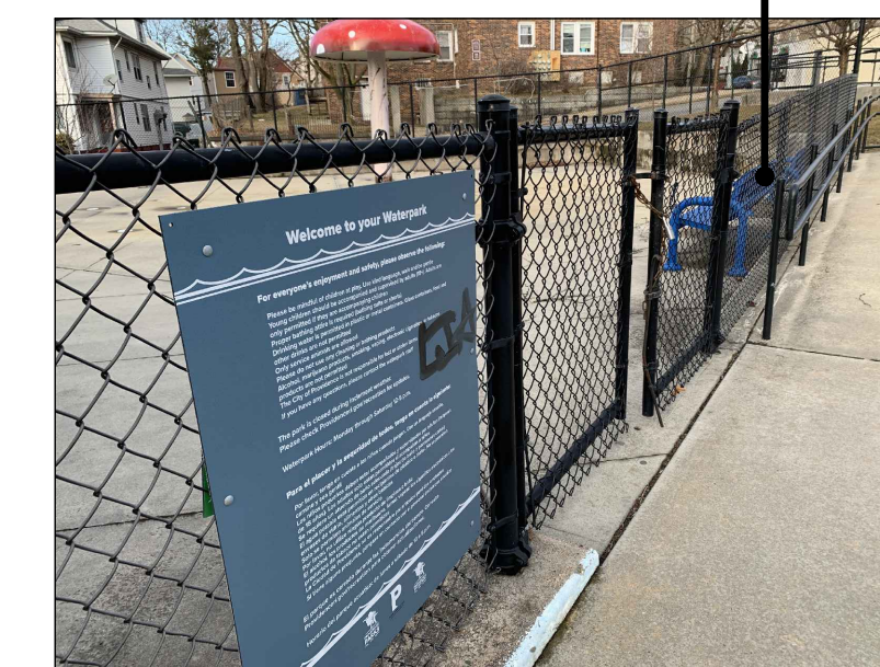
4 VIEW OF SERVICE GATE AT SPRAY PAD
