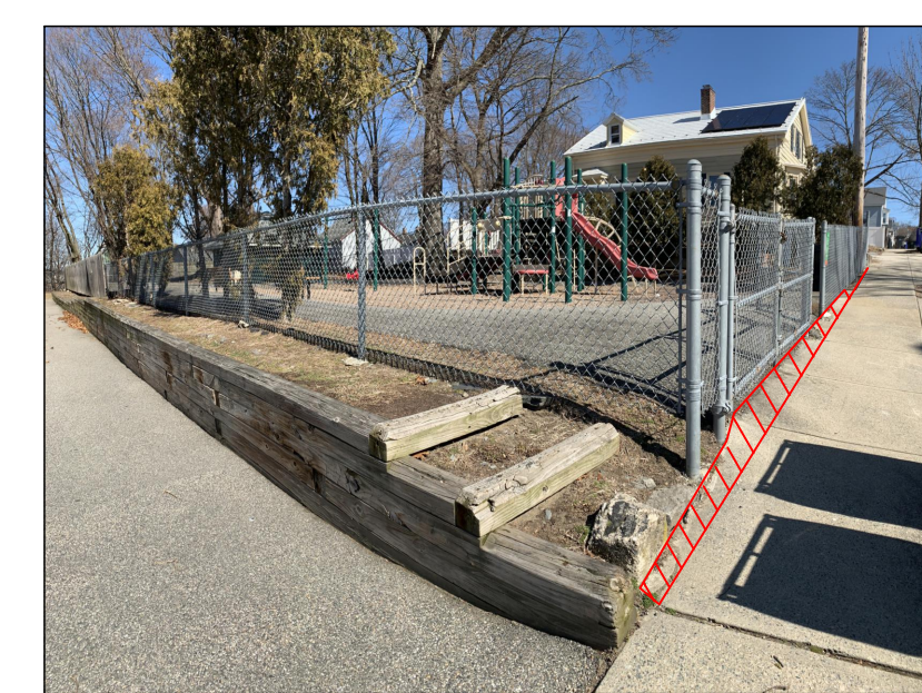
3 VIEW FROM PLEASANT ST AT SOUTHEAST CORNER
