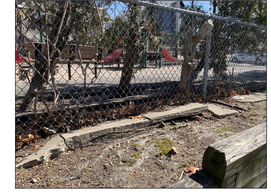
2 VIEW OF EX. RETAINING TO REMAIN AT SOUTH
