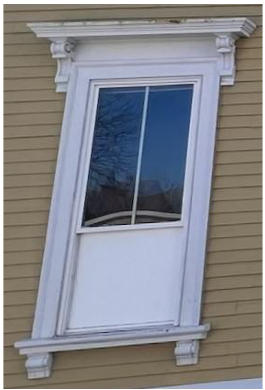
PHOTO OF EXISTING WINDOW
