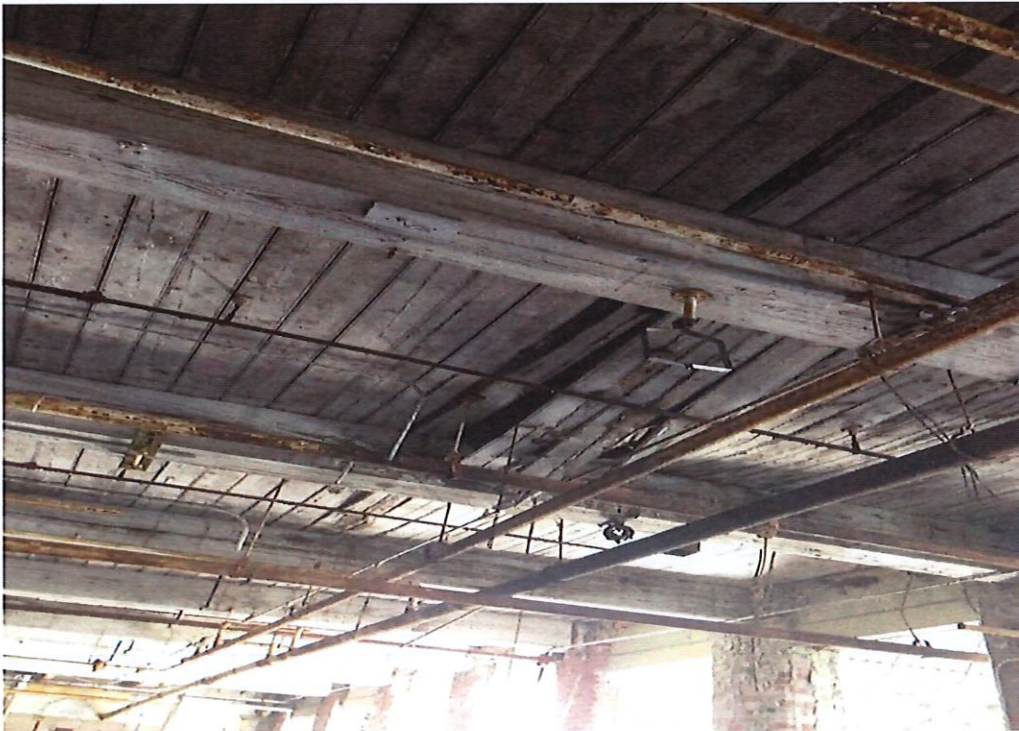
PHOTO 12: Typical Interior View of Second Floor Roof in Building 3
