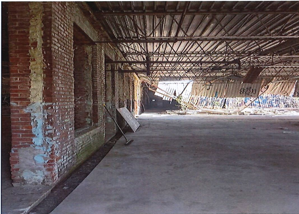
PHOTO 7: Interior View of Wall Between Buildings 2 and 3
