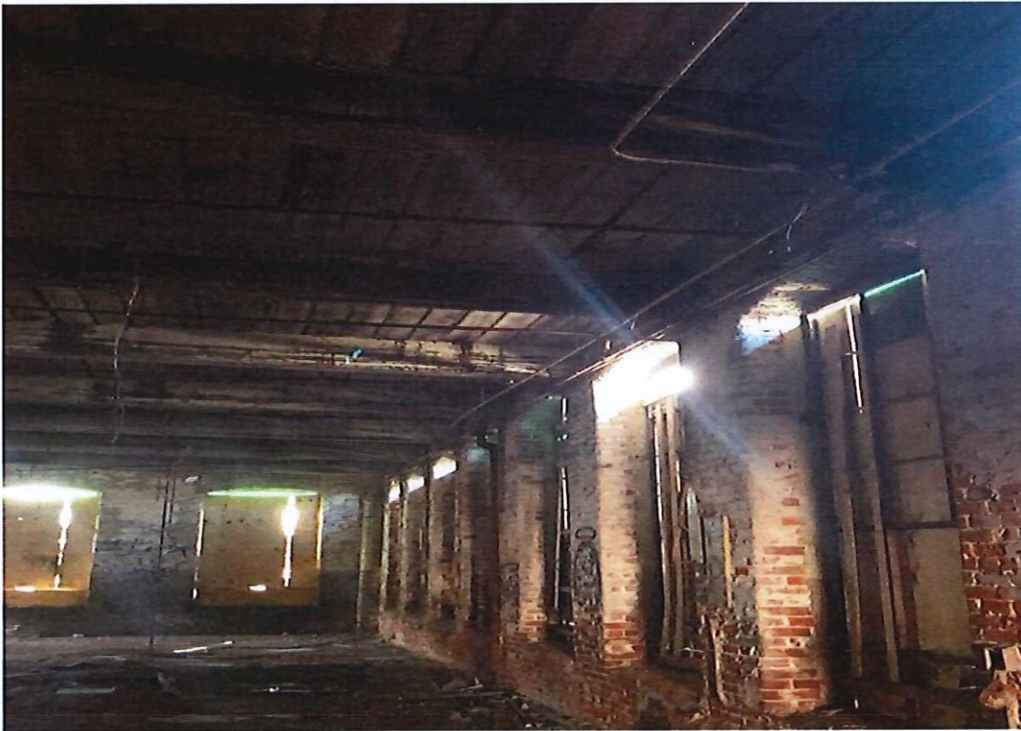
PHOTO 10: Typical Interior View of First Floor in Building 3
