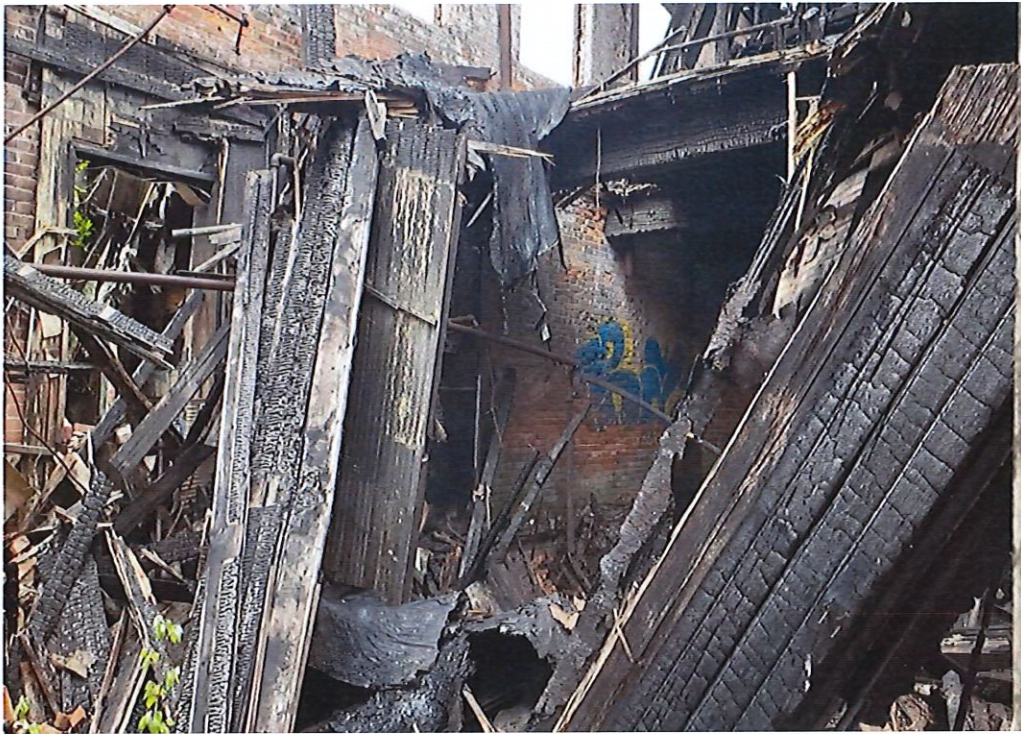
PHOTO 29: Typical Interior View of Building 8
