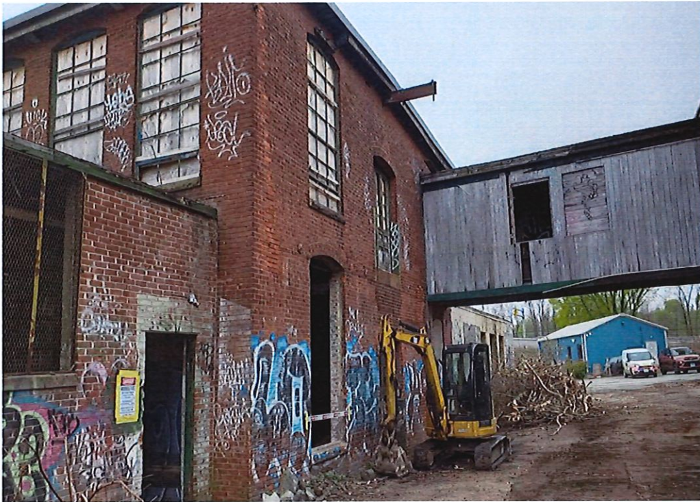
PHOTO 9: View of Western Face of Building 3
