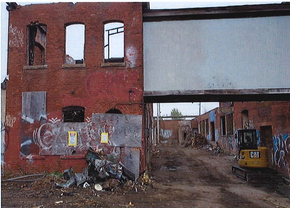
PHOTO 28: View of Southern Face of Building 8
