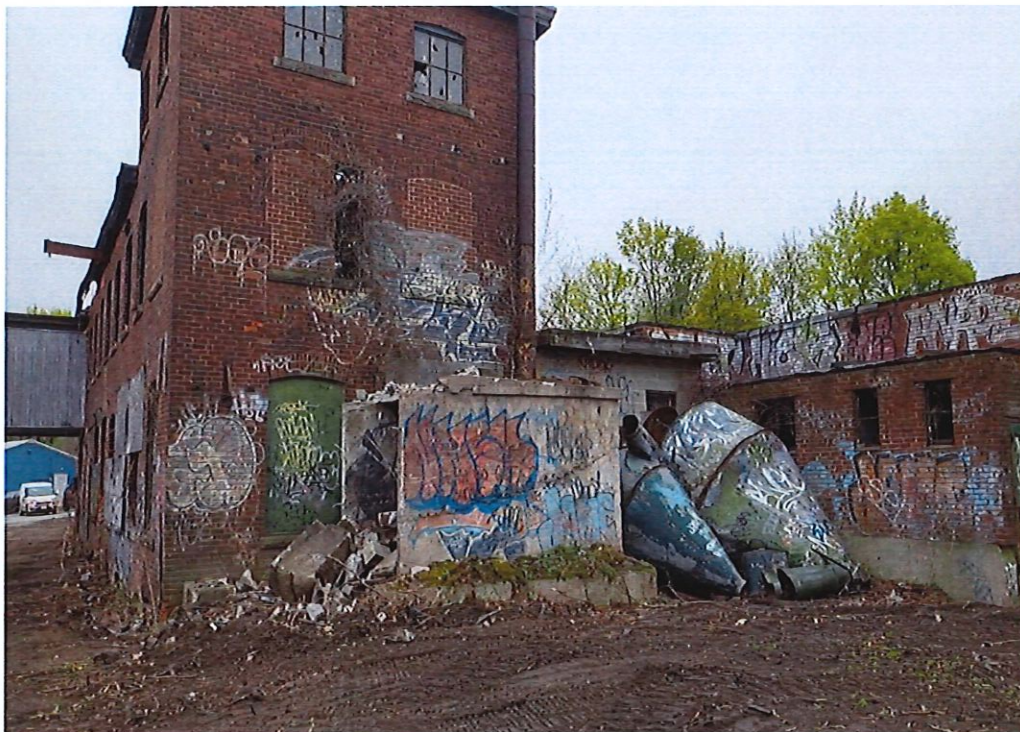
PHOTO 27: View of Northern Face of Building 8
