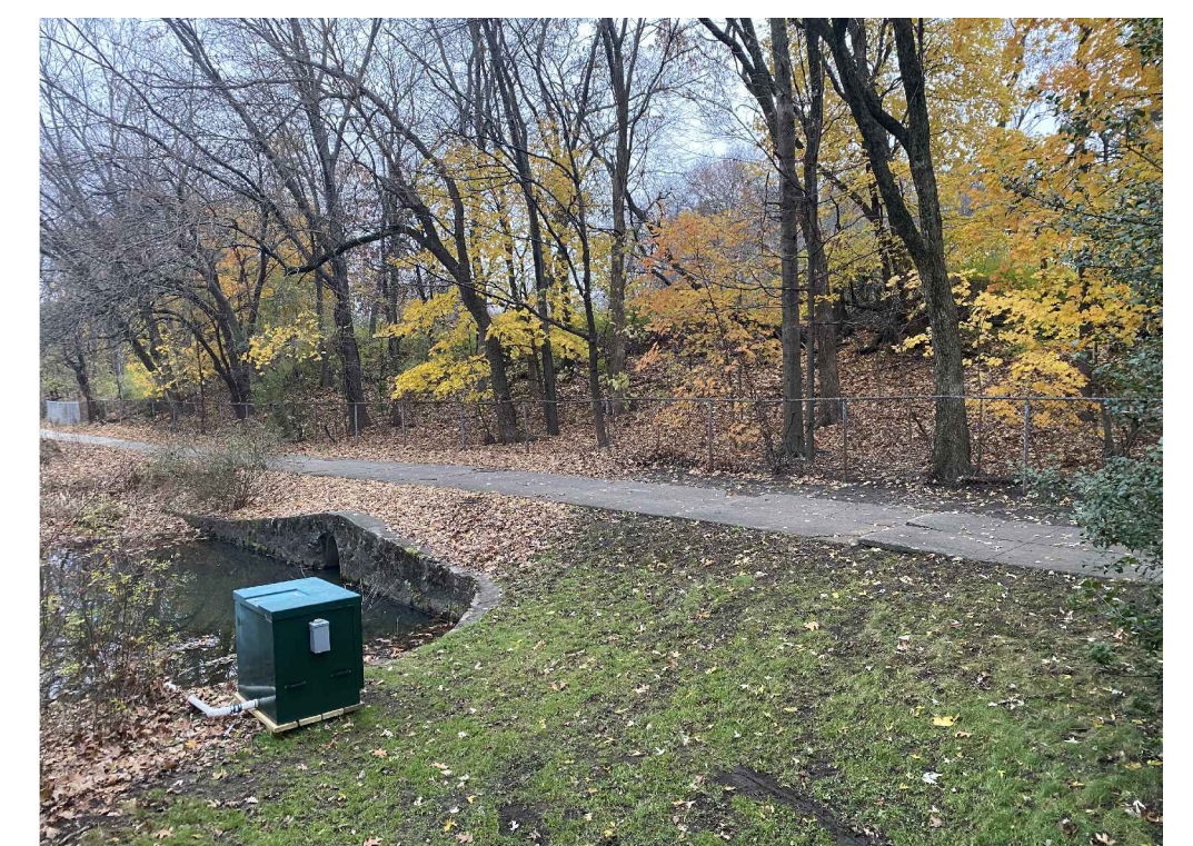
B. LOOKING SOUTHEAST TOWARDS PROJECT AREA
