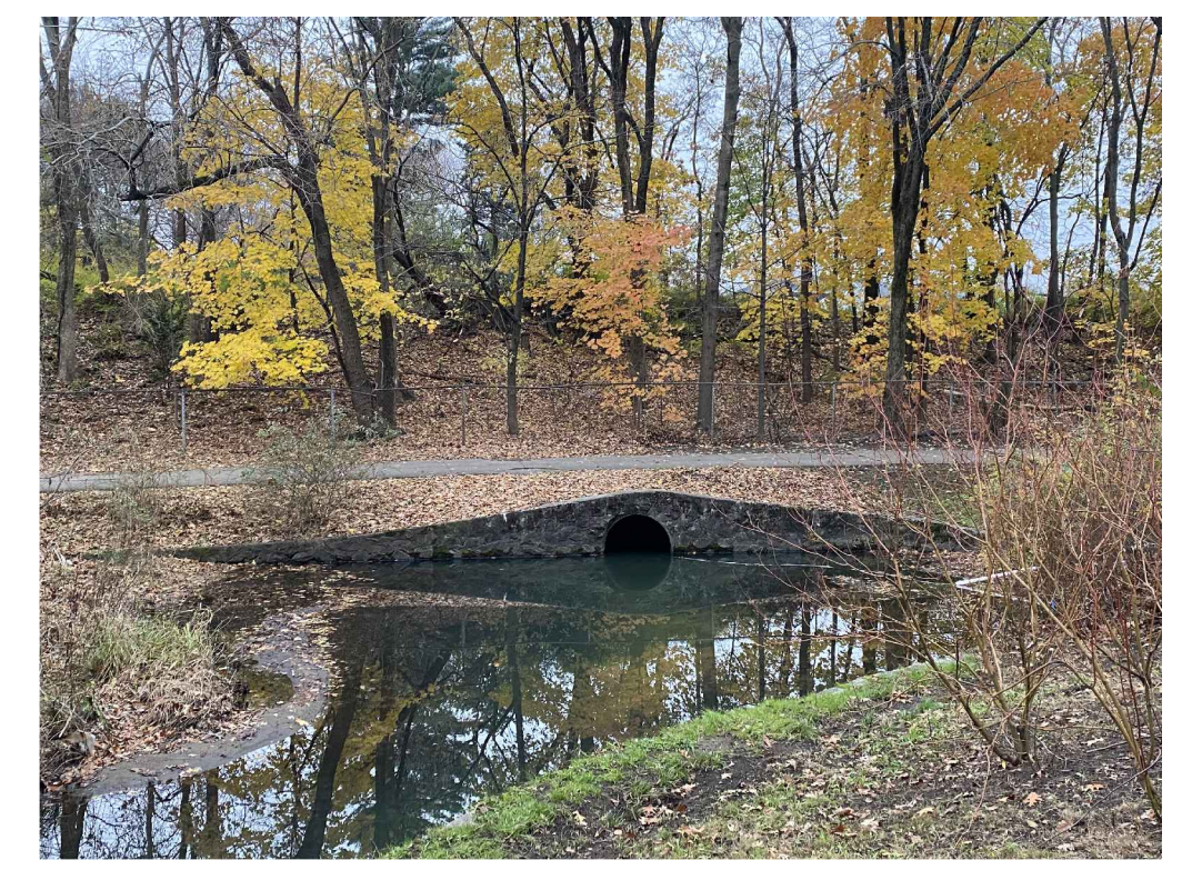
A. LOOKING TOWARDS EXISTING 48" OUTFALL
