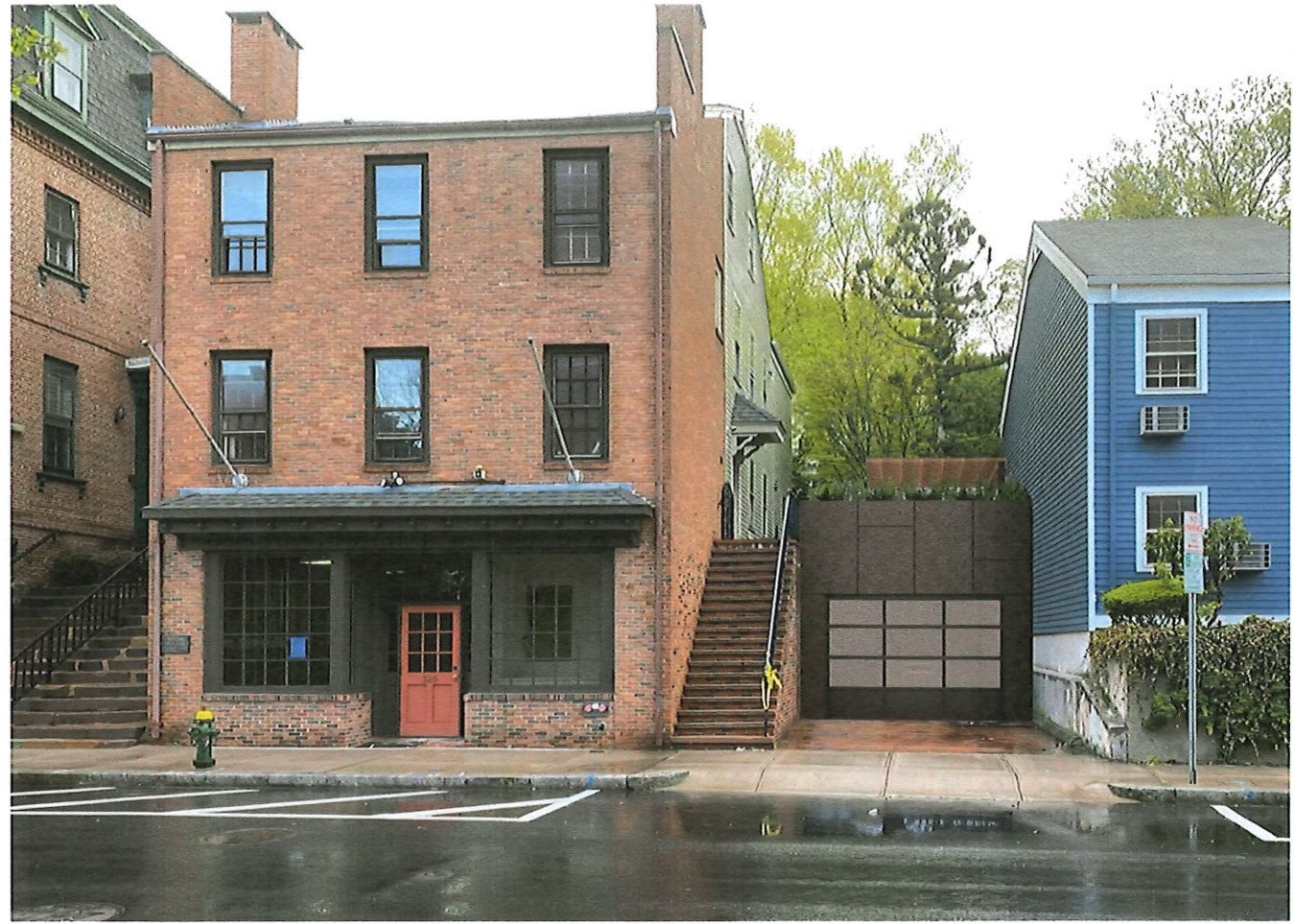
320 South Main Street with Proposed Garage and Painted Storefront
