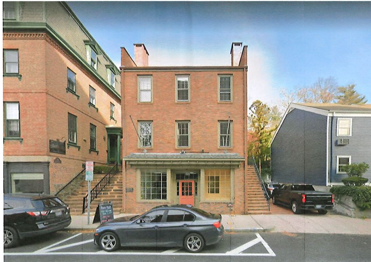
320 South Main Street Existing
