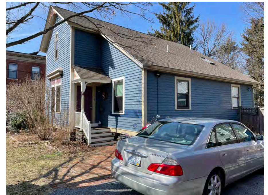
4 SOUTHEAST Photograph: 7 Gilbert St., Existing NOT TO SCALE
