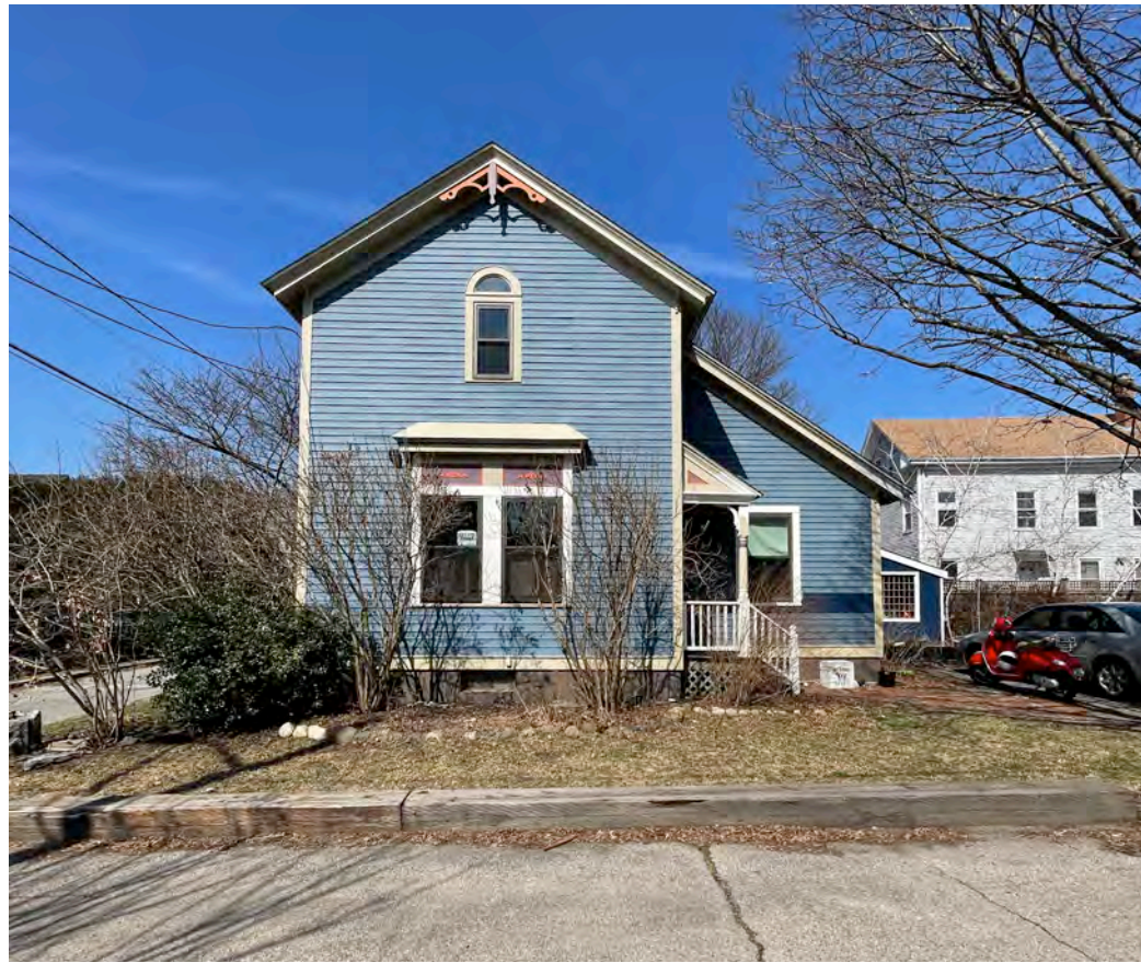
1 SOUTH Photograph: 7 Gilbert St., Existing NOT TO SCALE
