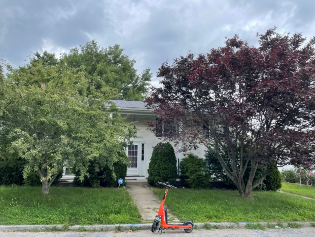
View from Liege Street
