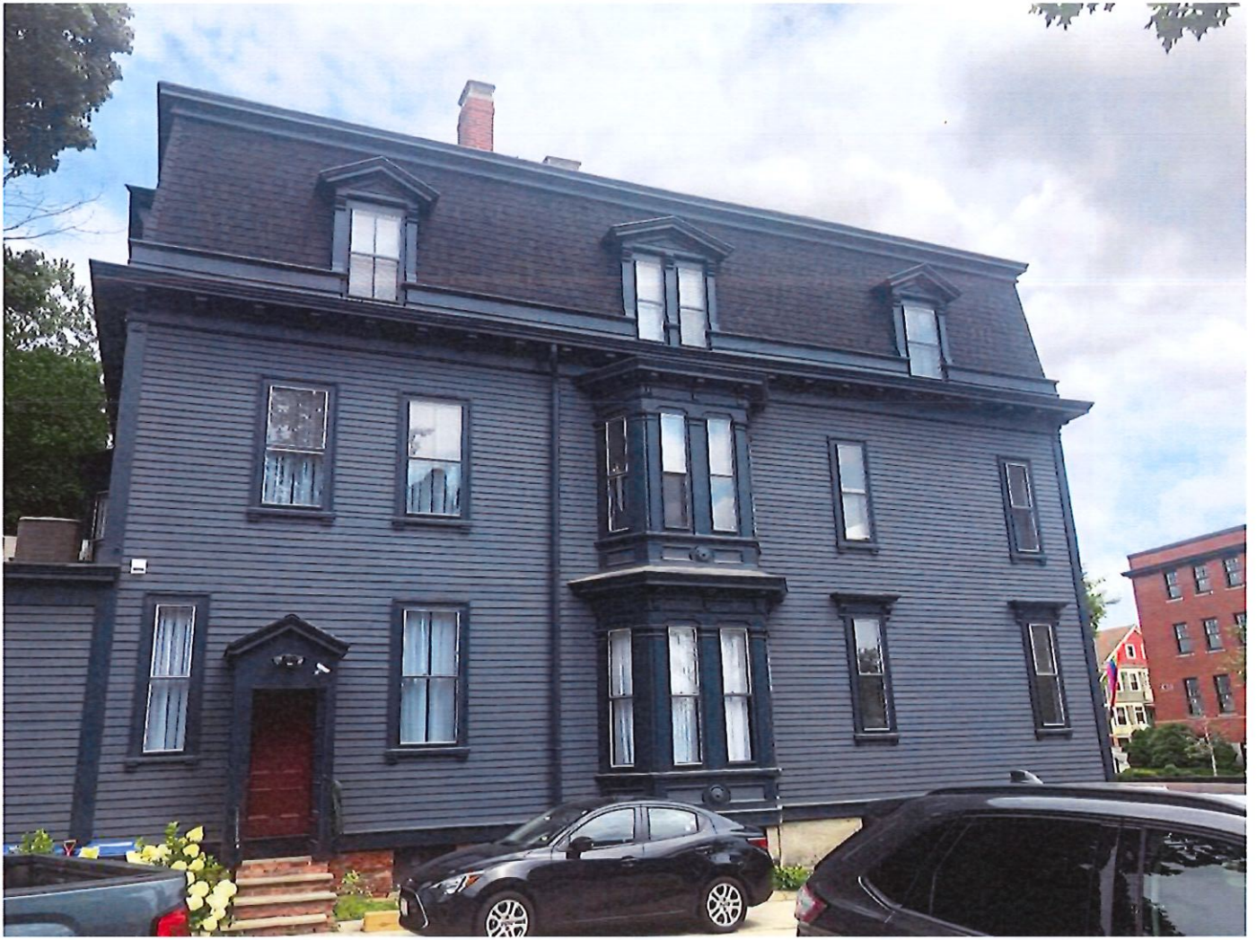
2 - 535 Broadway - west side to shared driveway
