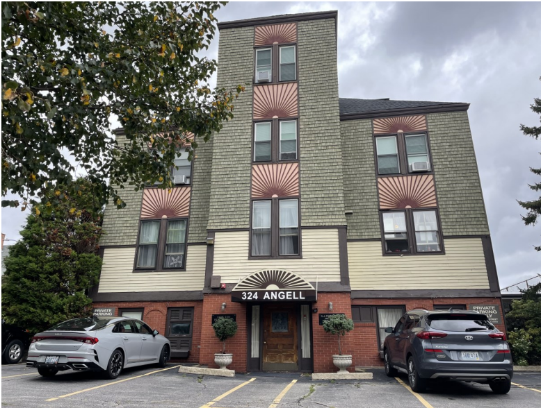
View of the house
