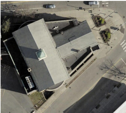
Aerial view of the building
