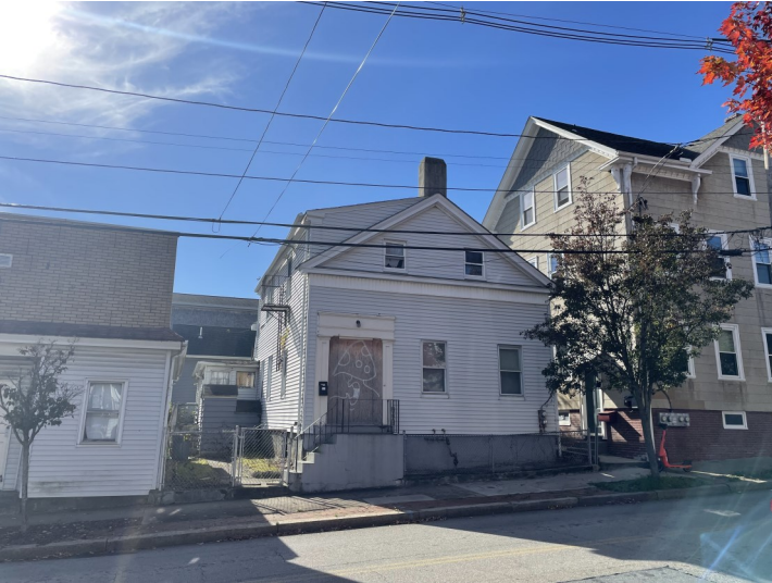
View from Douglas Ave
