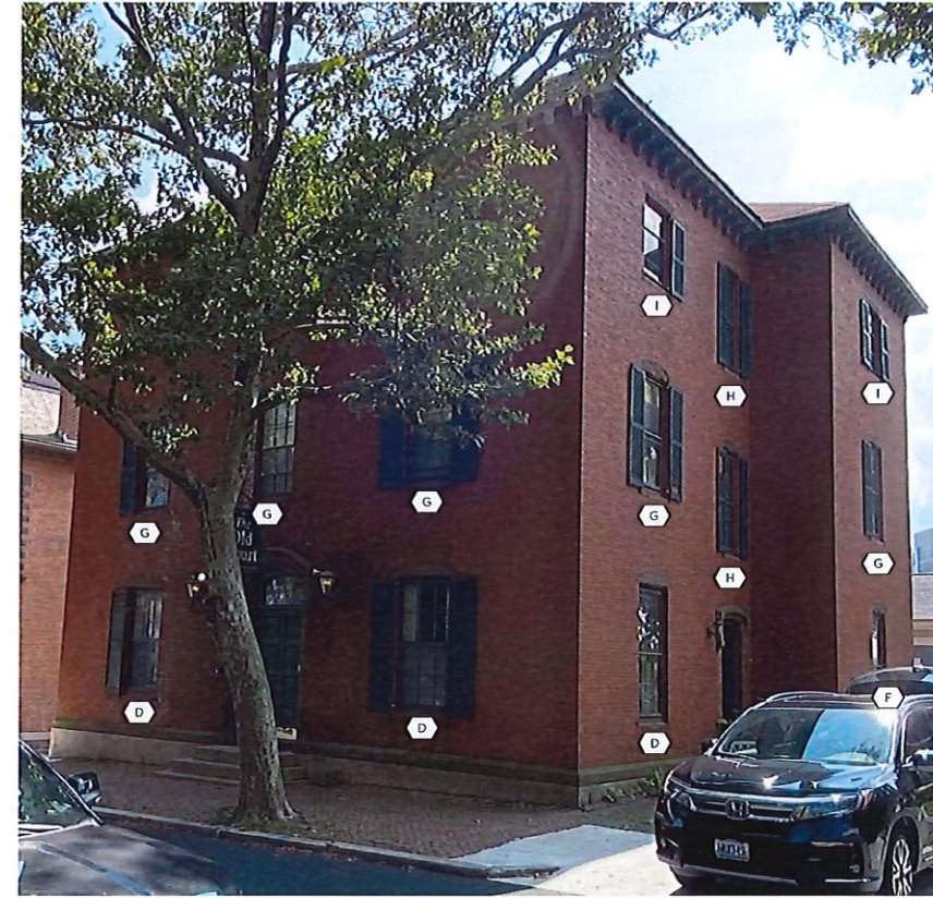
2 NORTH EAST CORNER (LOOKING SOUTH EAST FROM BENEFIT ST) DD.3
