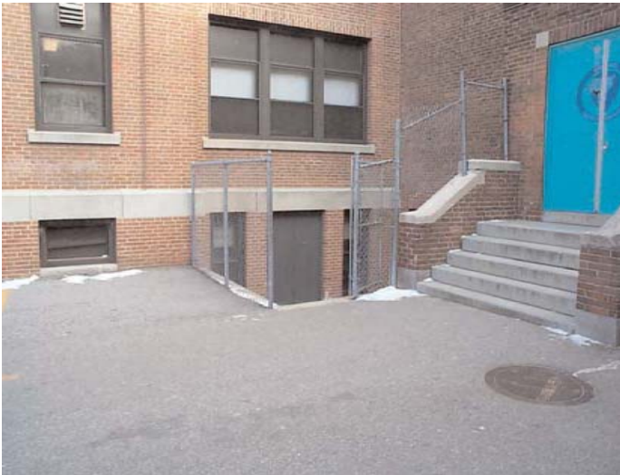
Side C, Doors 5 & 6 (Basement)
