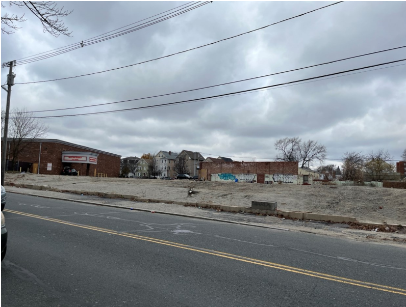
View of the building from Thurbers Ave
