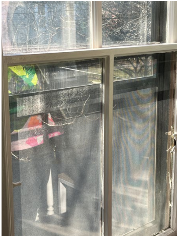
Figure 12 - sash replacement - Heritage
