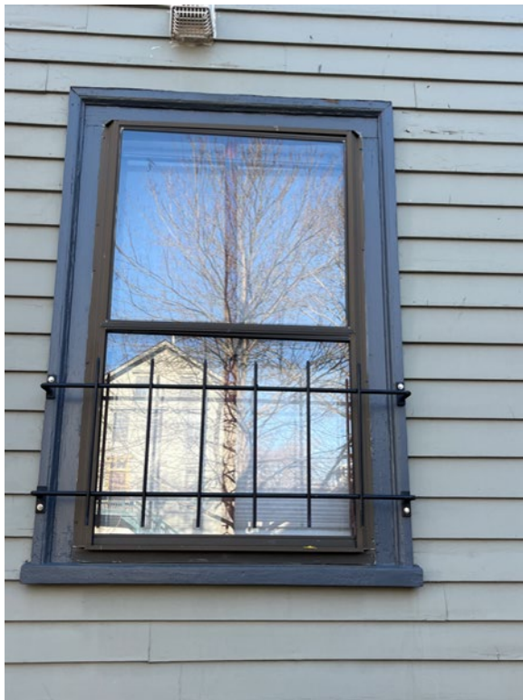
Figure 8 - Window "A" – Rear
