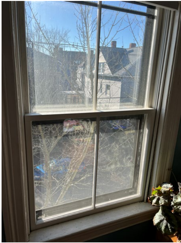
Figure 13 - Sash replacement – 5/8" muntin
