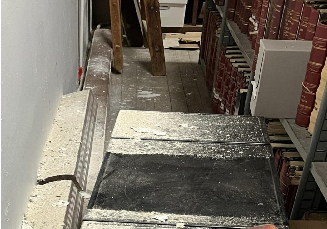
An accumulation of plaster dust on archival documents and shelves from continued deterioration of the City Archives' mezzanine walls.
