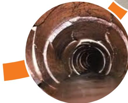
Cross-Contamination from Broken Sewer
