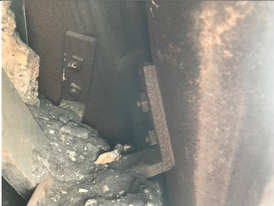
Figure 23. Comments: View of brackets securing decorative cast iron to structural steel roof framing. Note that there is no waterproofing or flashing installed where the clips penetrate the terracotta roof deck.
