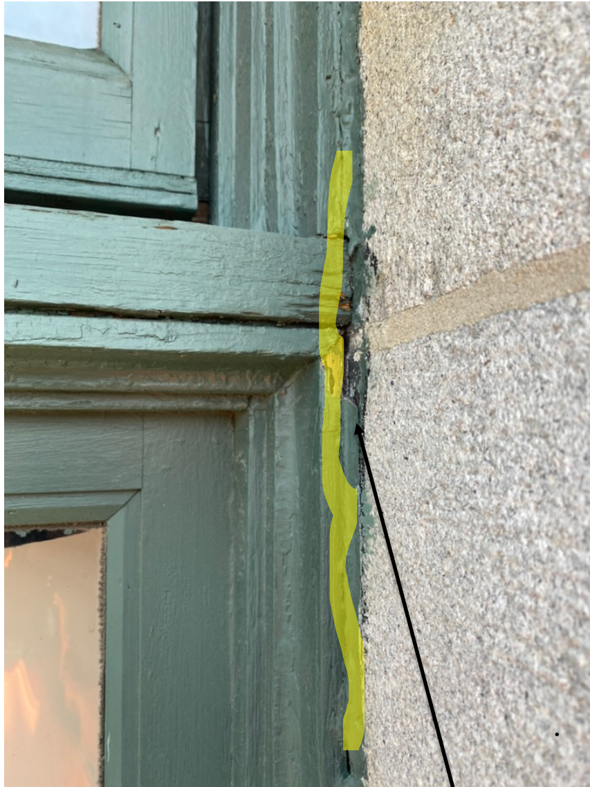
Photograph – 1: Photo depicts the typical application of asbestos caulk at the exterior window frames throughout the exterior of the Providence City Hall structure.
