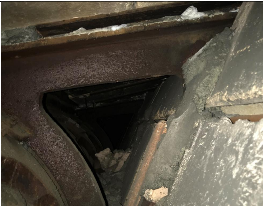
Figure 24. Comments: View of structural cornice support brackets and terracotta roof deck. Note that there is no waterproofing or flashing installed where the brackets penetrate the terracotta roof deck.
