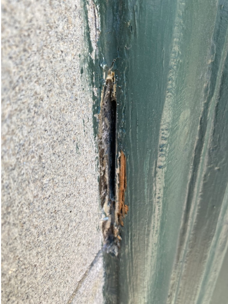
Photograph – 5: Photo depicts the typical location and application of asbestos caulk at the exterior window frames throughout the structure.
