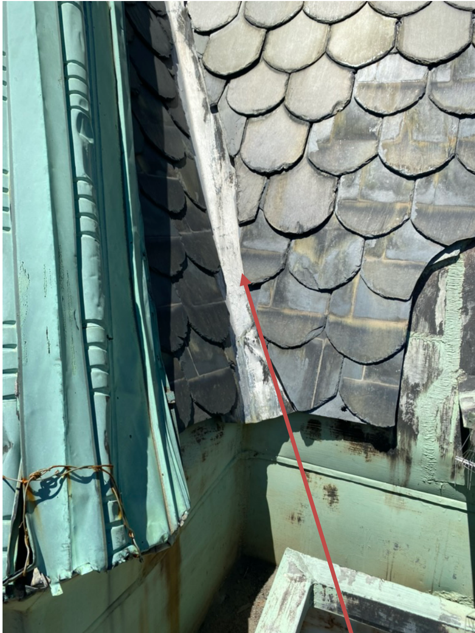
Photograph – 6: Photo depicts the typical application of asbestos roof paint at the exterior of the structure.
