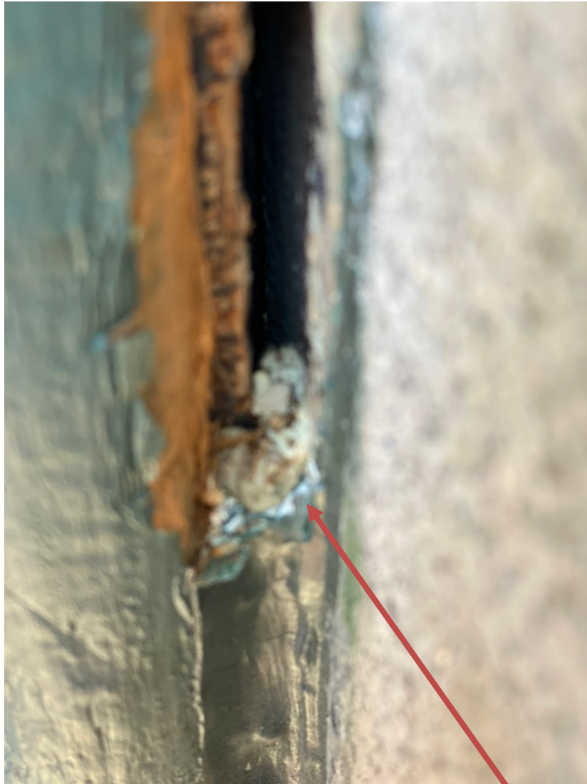
Photograph – 4: Photo depicts the typical location and application of asbestos caulk at the exterior window frames throughout the structure.
