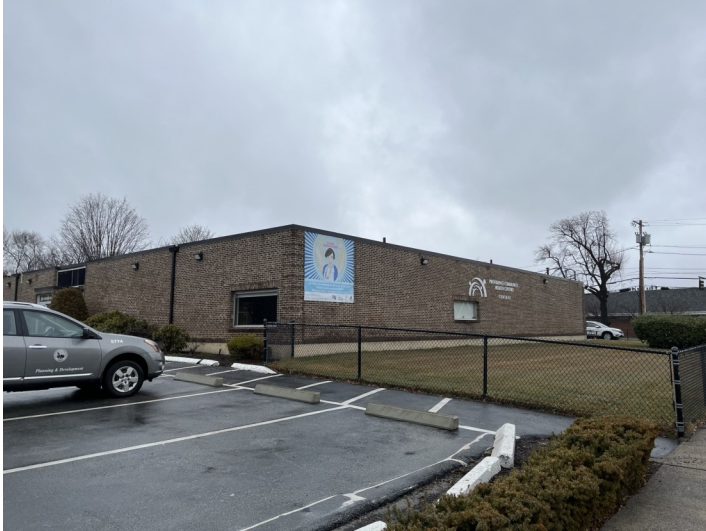
View of the building from Cranston Street
