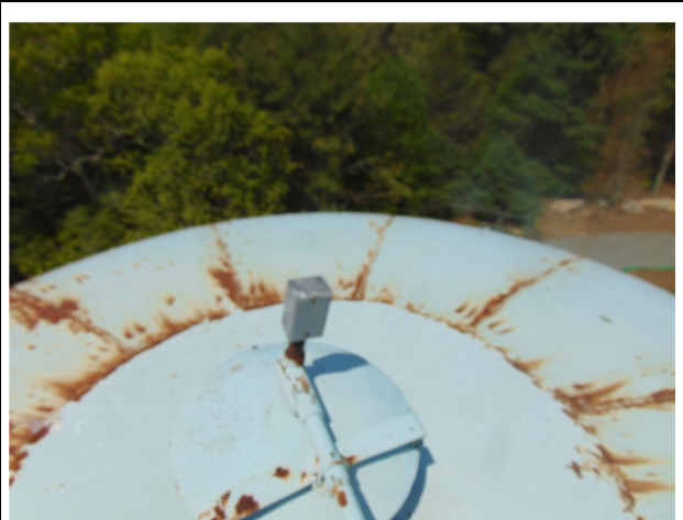
16) 16-Typical condition of roof and vent overview
