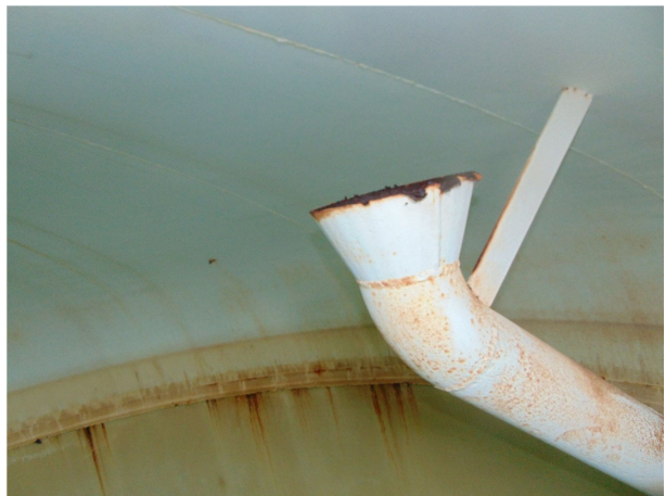
20) 20-Overflow weir funnel
