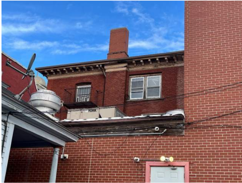
Figure 7 - south wall, third floor
