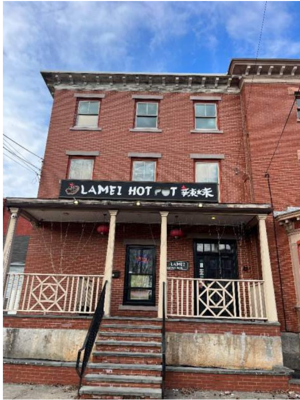
Figure 3 - East wall - 2000 addition
