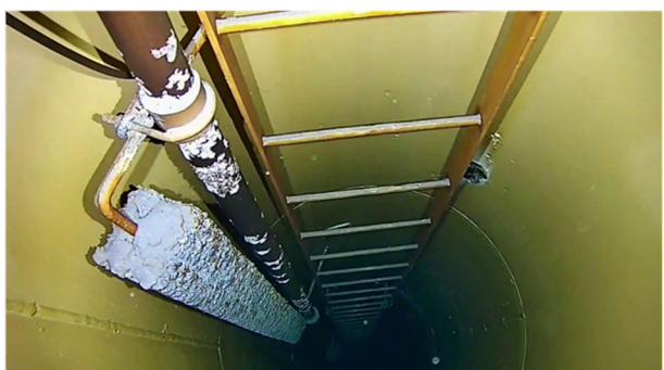
29) 6:32-Interior of riser pipe
