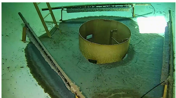
28) 5:47-Riser pipe opening and anode overview
