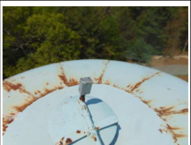
16) 16-Typical condition of roof and vent overview
