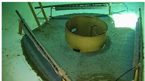
28) 5:47-Riser pipe opening and anode overview
