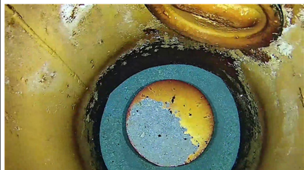
31) 8:18-Bottom of riser pipe with inlet/outlet
