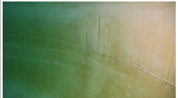
25) 3:30-Intact coating on lower shell
