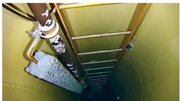
29) 6:32-Interior of riser pipe
